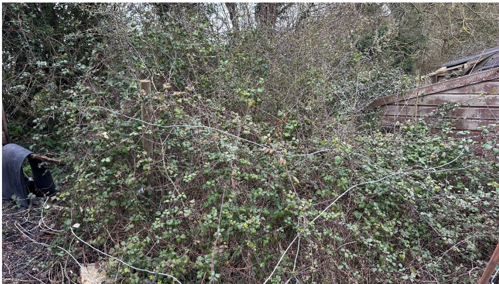
Plate 8: Scrub surrounds the stable building.
