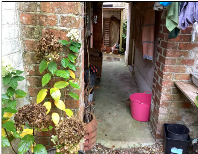
SVP1 location to manhole 1
