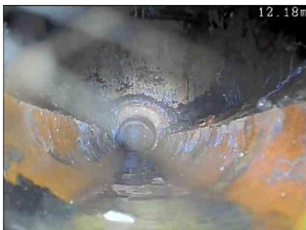
MH2X_7163d9a0-2a58-4bde-a1a9-9803b54bf5ee_20241121_120350_978.jpg, 00:01:28, 12.18 m General observation, Enters MH3
