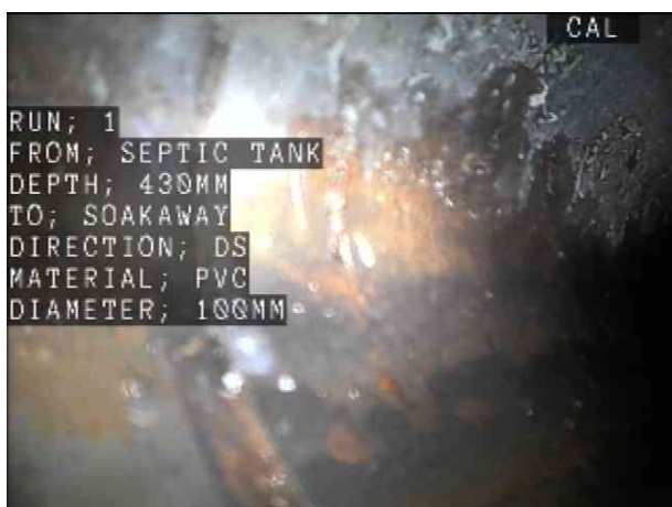
SepticTankX_4ff9bda3-935c-4713-8895-a2852ad849cd_20241121_114056_807.jpg, 00:00:00, 0.00 m Start of survey
