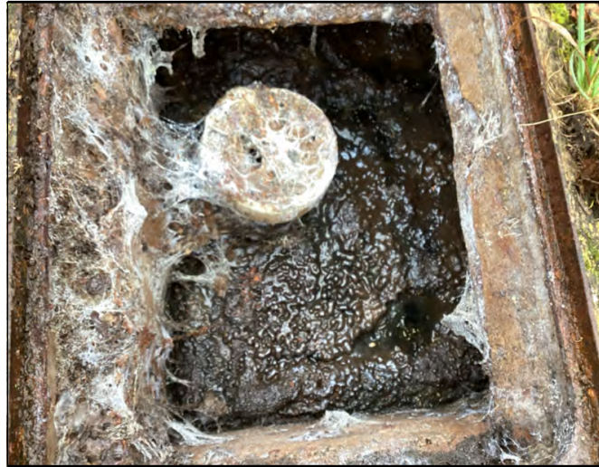
septic tank chamber 1 on arrival
