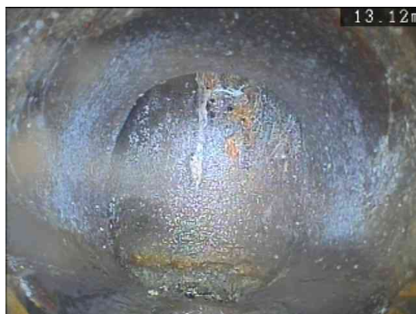
MH2X_b72b9686-9c99-458a-8f6d-dc915f3b60c3_20241121_120518_713.jpg, 00:01:32, 13.12 m Finish survey, Reached inlet to septic tank
