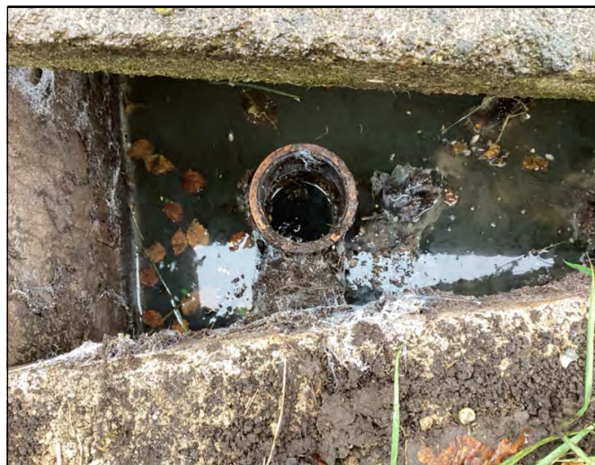
septic tank chamber 2 on arrival
