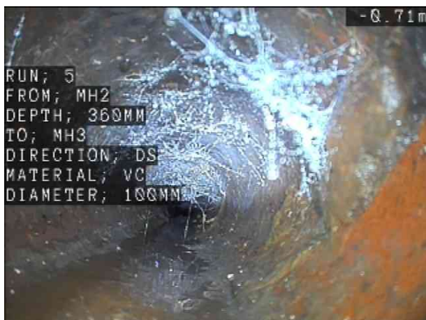
MH2X_0e280976-1d7b-4a46-a9b6-f66c632bf85d_20241121_120010_936.jpg, 00:00:00, 0.00 m Start of survey
