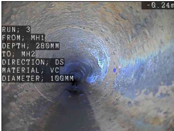
MH1X_4d6969ac-2977-467d-9507-78f824289f0a_20241121_1 14934_886.jpg, 00:00:00, 0.00 m Start of survey
