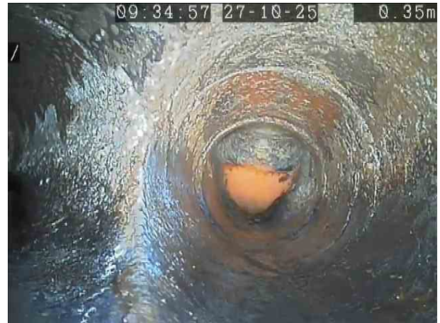
1c8a0ad6-aeab-4bb6-9fd2-4ac4f40f7d13.png, 00:00:24, 0.35 m Junction at 10 o'clock, 100mm dia
