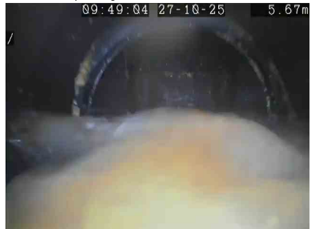
222b057b-f4ca-4d2e-97e3-92ab29034af7.png, 00:01:59, 5.67 m Finish node, manhole, reference: I/C3 BURIED
