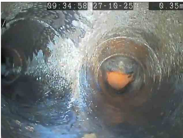
fdbf41fb-321d-4a69-baa3-74e95a19d159.png, 00:00:25, 0.35 m Line deviates left
