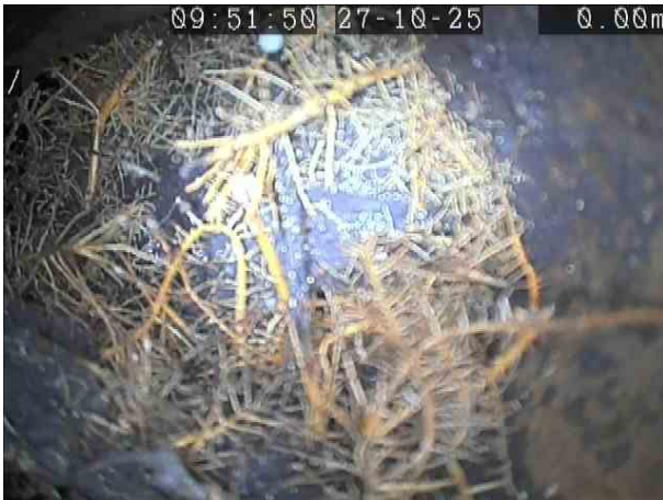
eb2104d7-7e24-4207-b4a1-63060fa71da8.png, 00:00:07, 0.00 m Start node, manhole, reference: DC
