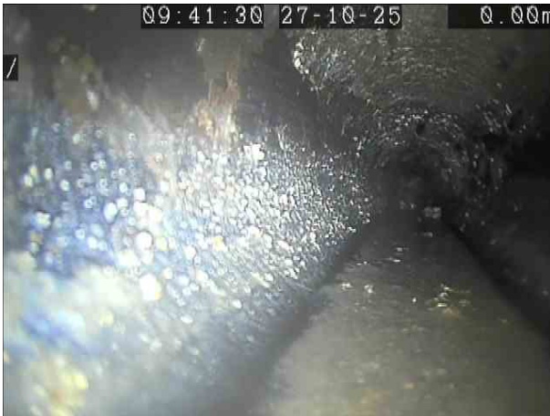
98d76d57-c896-48d3-9886-c05b168a7194.png, 00:00:10, 0.00 m Start node, manhole, reference: MH4
