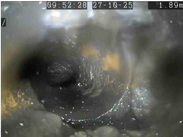
cf23fff4-fcc7-4db6-99b7-12f25f3ce381.png, 00:00:44, 1.89 m Line deviates left
