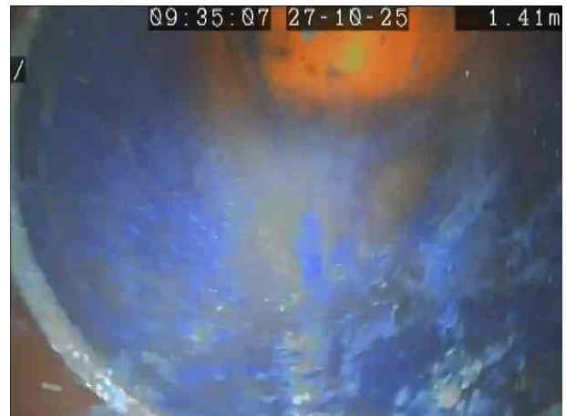
50fdef2b-6cfa-4c52-9996-b7f7f37fb40f.png, 00:00:33, 1.41 m Line deviates up
