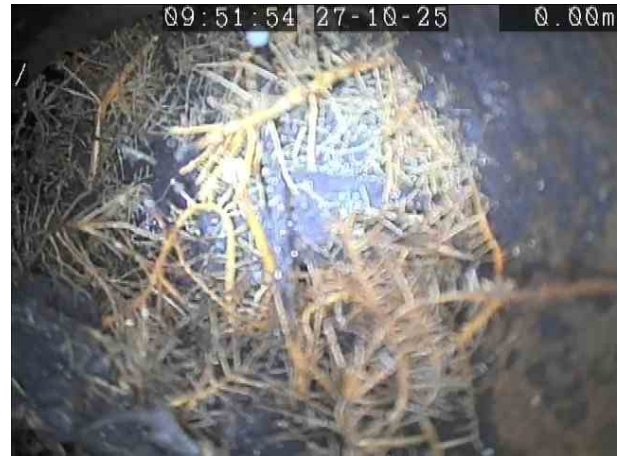
a465fbca-864e-420a-ad48-71e227b3eb67.png, 00:00:11, 0.00 m Roots, mass, 90% cross-sectional area loss
