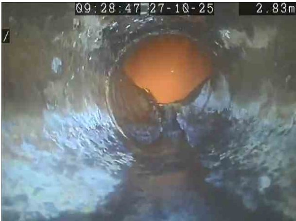
81f02555-0d89-468c-ae4f-4796d978f216.png, 00:00:32, 2.83 m Line deviates up
