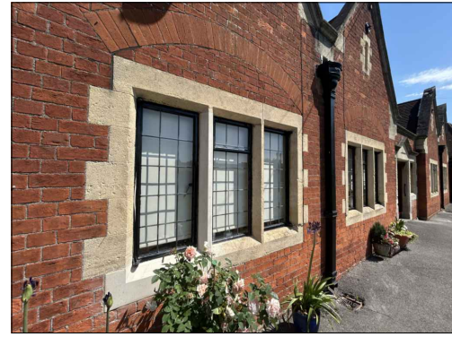
PHOTOGRAPH 4 Type 2 window (Replacement 1950s/60s metal single glazed leaded lights)
