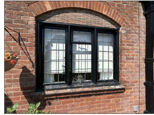
PHOTOGRAPH 3 Type 1 window (Timber frame with metal single glazed leaded lights)
