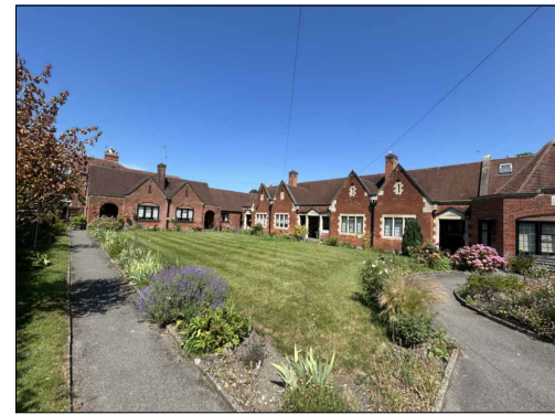
PHOTOGRAPH 1 East and South elevations
