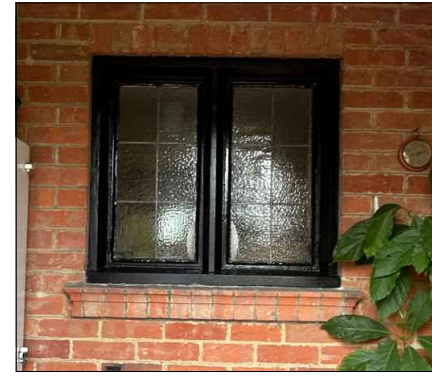
PHOTOGRAPH 5 Type 3 window (Replacement timber single glazed leaded lights)
