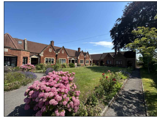
PHOTOGRAPH 2 West and South elevations
