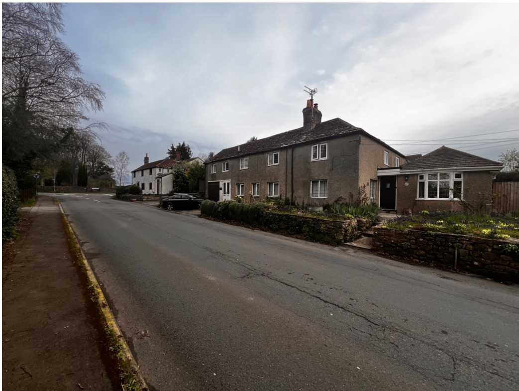
Circa 19 th C properties opposite Lydiard Farm – Rendered walls, natural and recon stone, slate and pantile roof finishes with uPVC windows. Properties have been significantly extended during the 20th century. Note these properties are elevated significantly above the road level.
