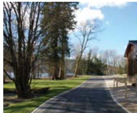
Fallbarrow Park, Windermere: Completed CellWeb TRP® Installation
