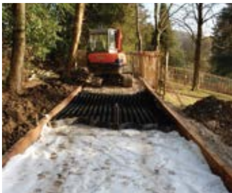
Fallbarrow Park, Windermere: CellWeb TRP® Installation
