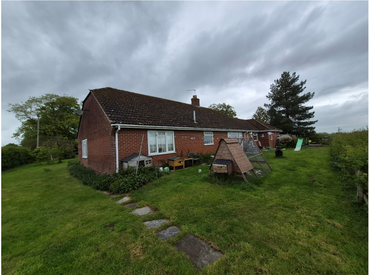
Southern elevation and rear
