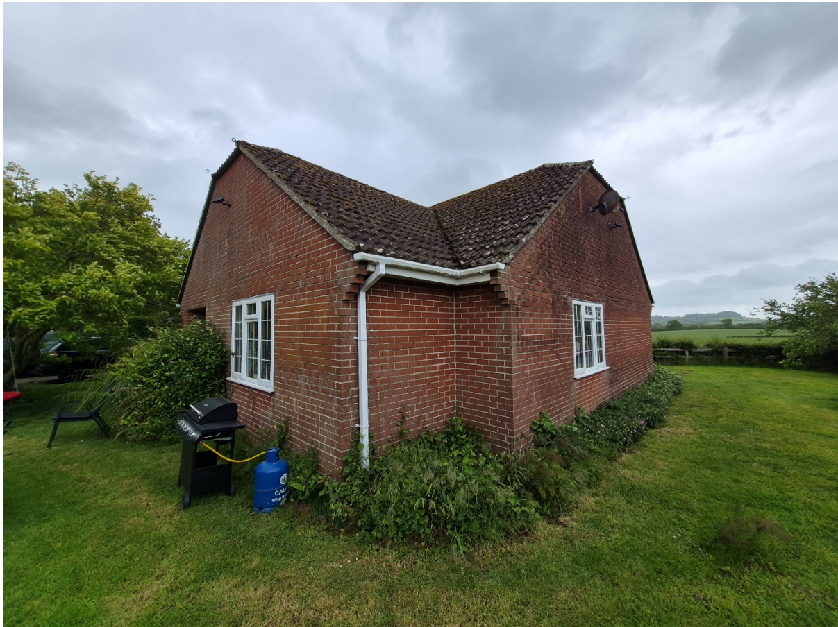
Southern elevation and front
