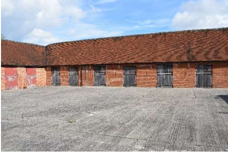
Fig8 Existing Barn Cii from courtyard (looking NE)
