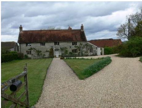
Fig4 Existing farmhouse from track
