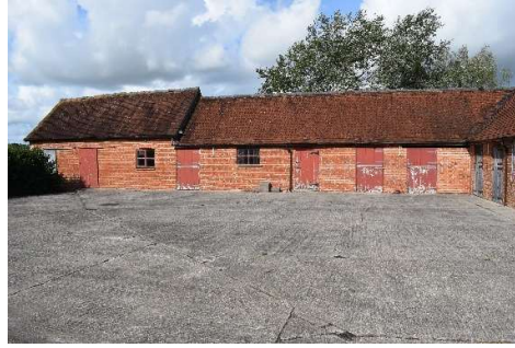
Fig9 Existing Barn Ci from courtyard (looking NW)
