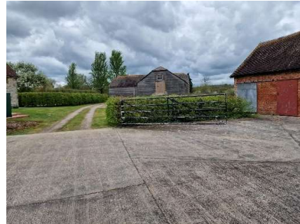
Fig7 Existing Barn B showing relation to Barn C and farmhouse
