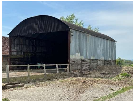
Fig11 Existing Dutch barn from the East
