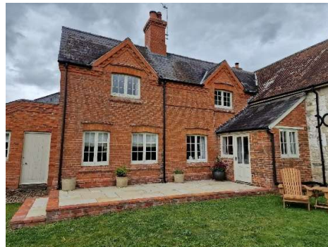
Fig5 Existing farmhouse from rear garden
