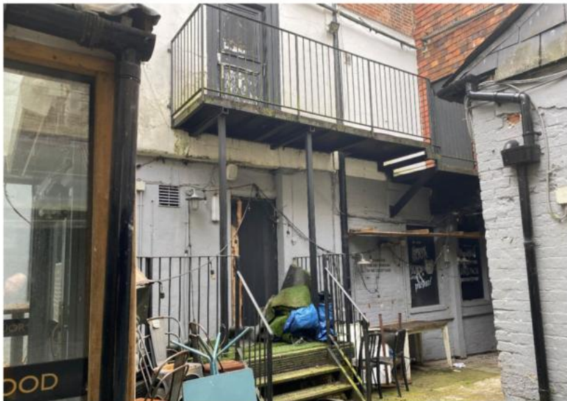
Figure 12: The southern yard, Blue Boar arch on the right.
