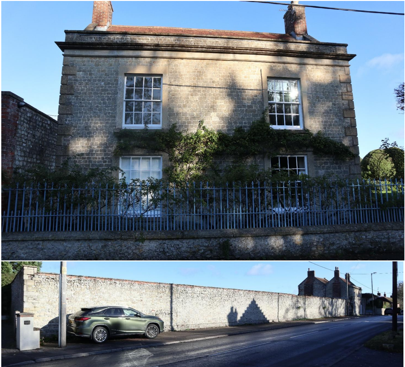
Figure 3 The Cotes (Grade II) two storey house (above) and the attached Boreham Road boundary wall to west (below)
