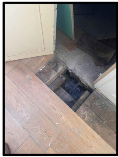
PHOTO 1 - GROUND FLOOR INVESTIGATION BENEATH NEWEL POST
