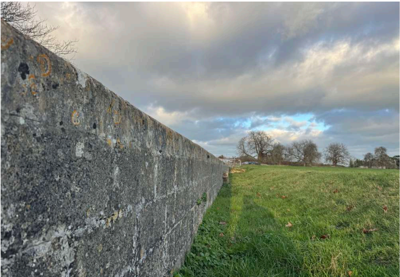
Figure 3.9: Modern concrete ha-ha forming southern garden edge
