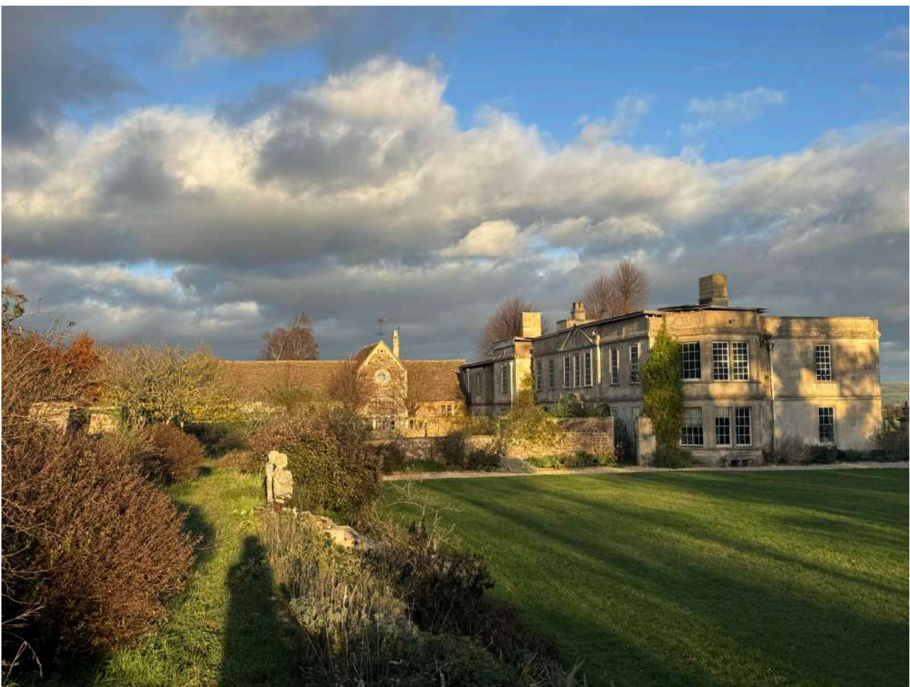
Figure 3.8: Raised terrace within Larch Garden
