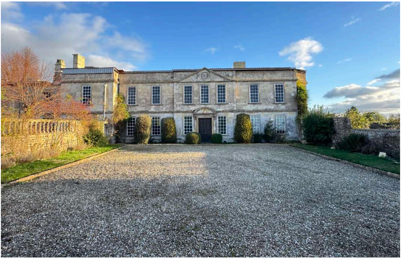
Figure 3.4: North approach and courtyard
