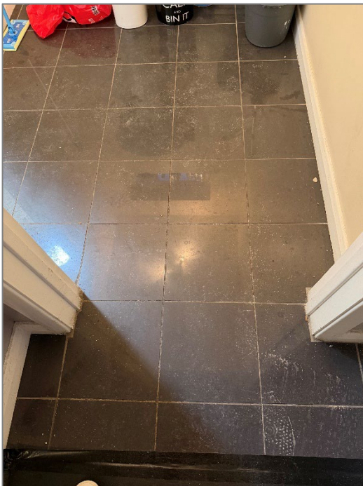
Figure 21 - Modern floor tiles at ground floor
