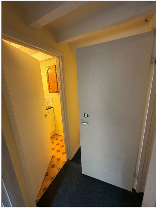
Figure 23 - Existing vinyl flooring
