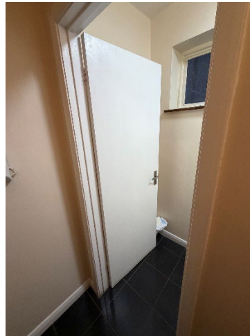
Figure 7 - Ground floor door 2
