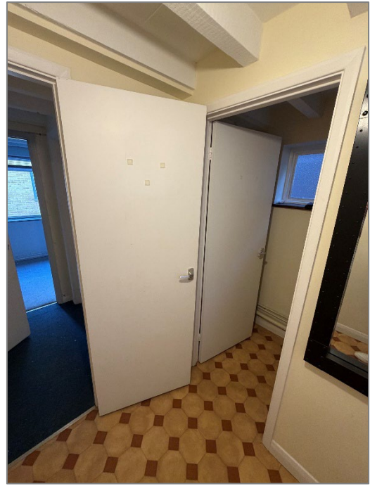
Figure 24 - Existing vinyl flooring
