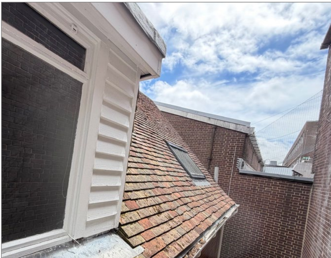
Figure 5 – Existing roof eastern elevation
