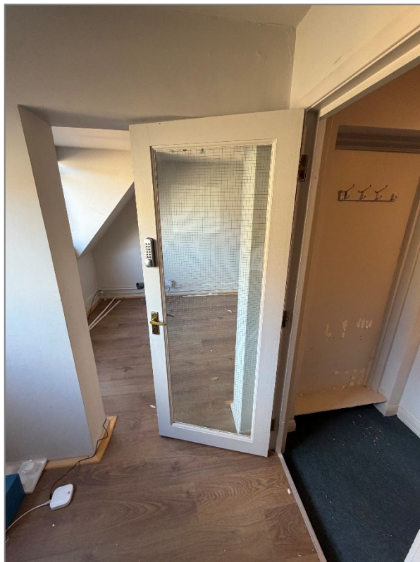
Figure 27 - Second floor wood vinyl flooring
