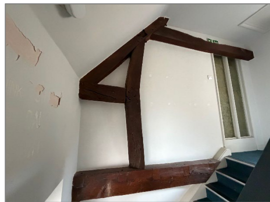
Figure 4 - Positioning of existing exposed beam on stairwell
