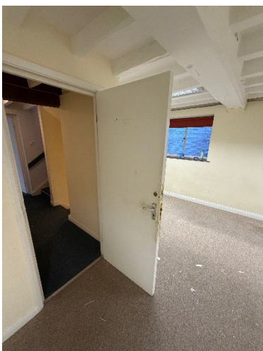
Figure 12 - First floor doors
