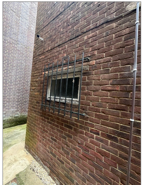
Figure 18 - Existing brickwork on south elevation
