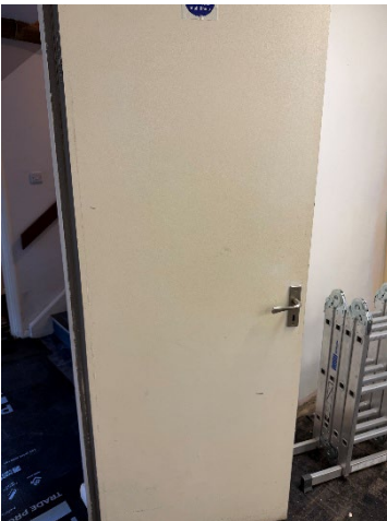
Figure 9 - Ground floor door 4
