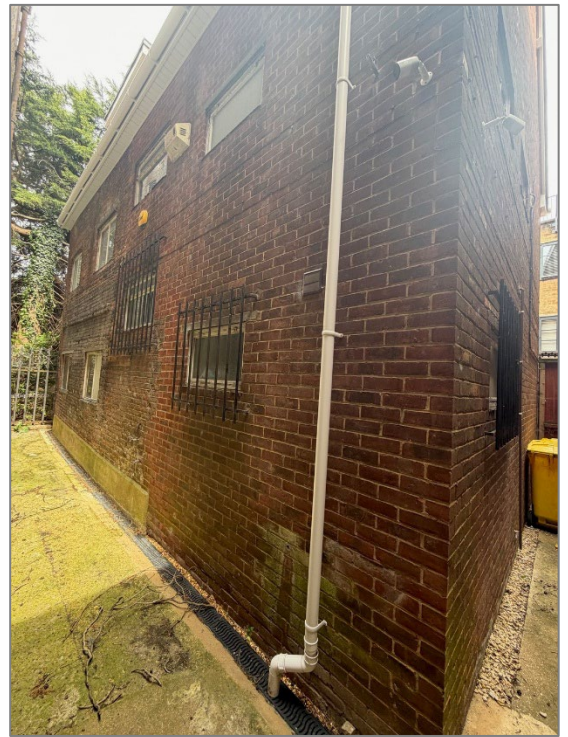
Figure 16 - Existing brickwork in good condition
