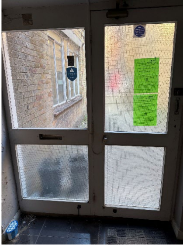
Figure 6 - Ground floor door 1
