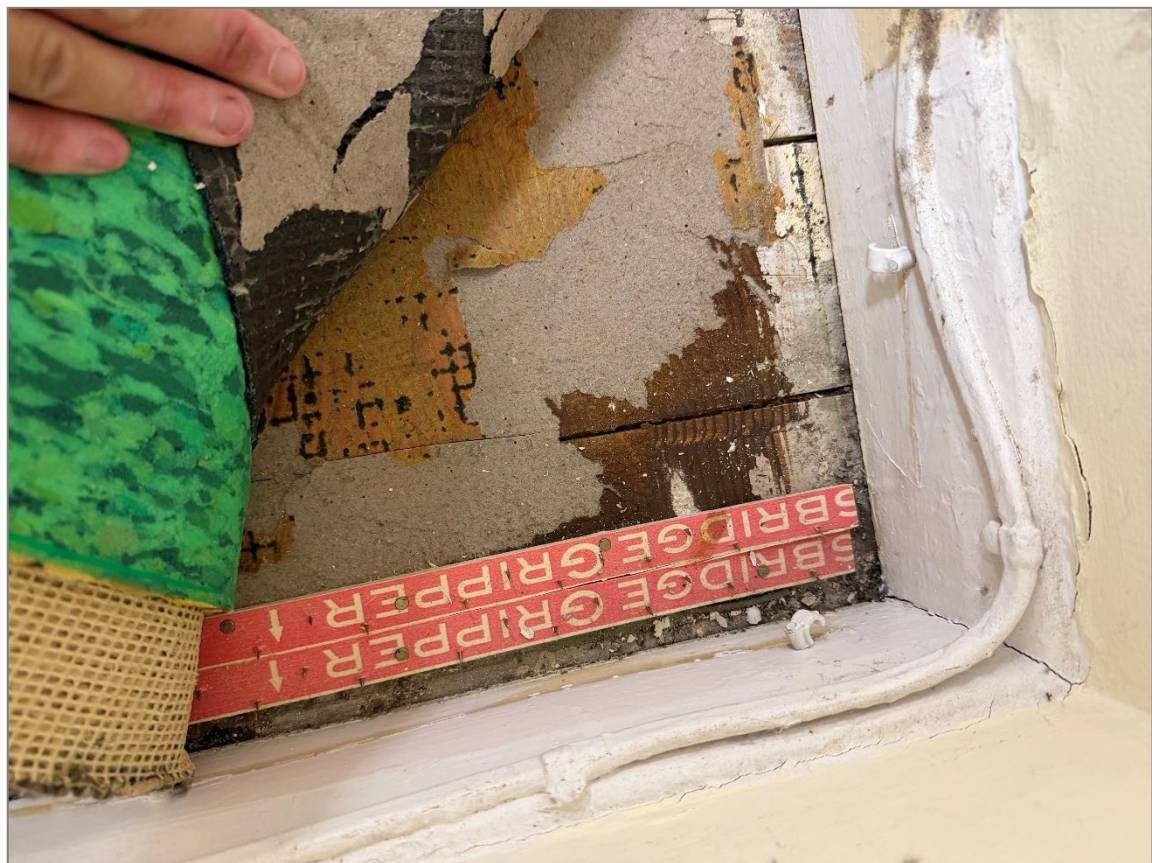
Figure 25 - Existing floor boards at first floor
