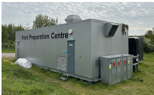
Example of Paint Booth enclosure located within yard area, constructed of prefinished metal panels colour Goosewing Grey (RAL 08 07 005)
