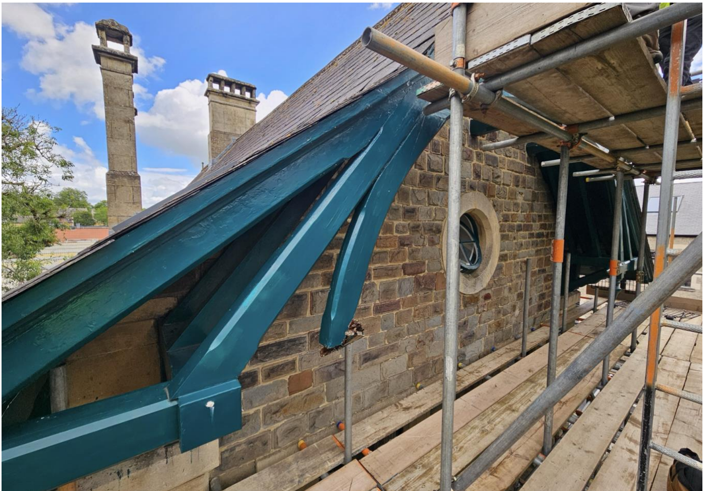
Fig.1: Bank House South West Elevation Gable
