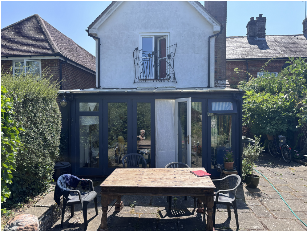
EXISTING CONSERVATORY, THIS ON THE NON LISTED PART OF THE PROPERT AS EXTENDED S/2003/0817
