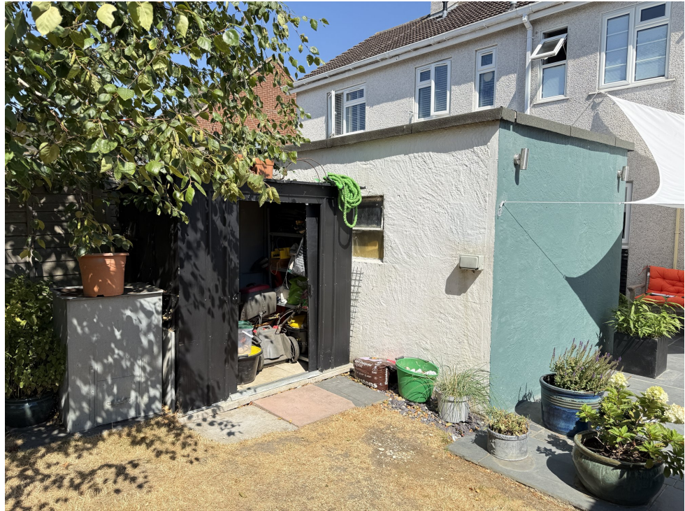
Figure 7 – Existing outbuilding, rear elevation
