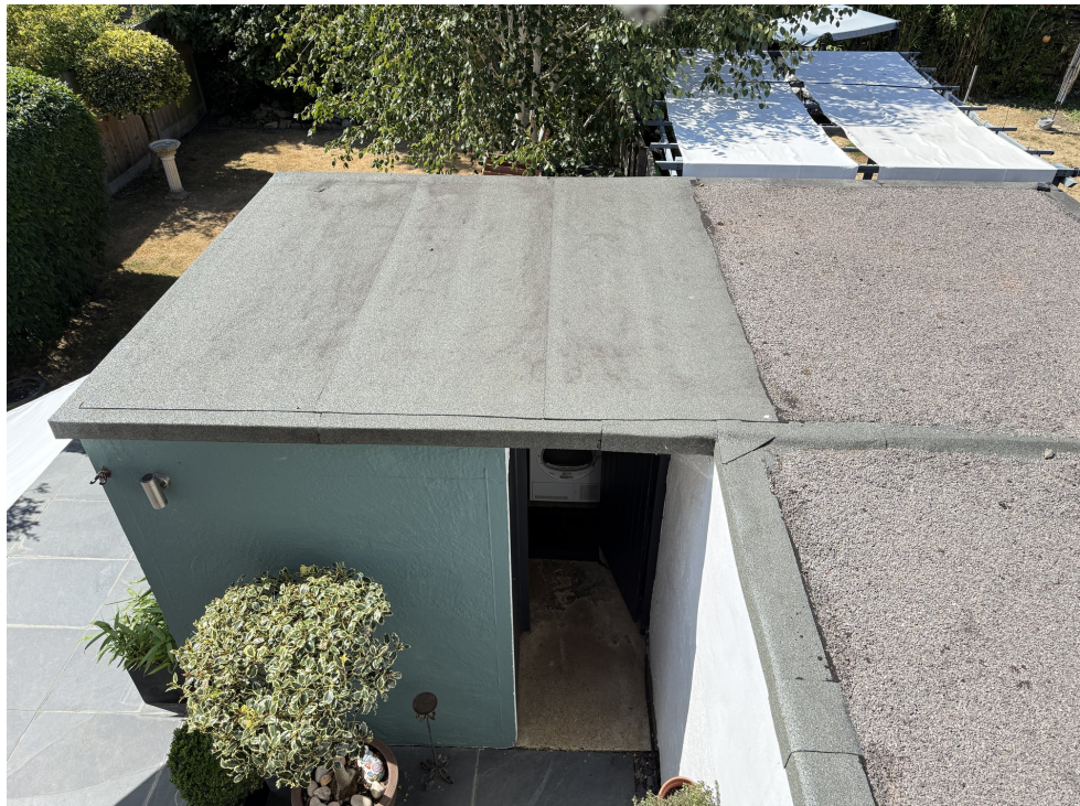
Figure 8 – Existing outbuilding showing roof, entrance and boundary
