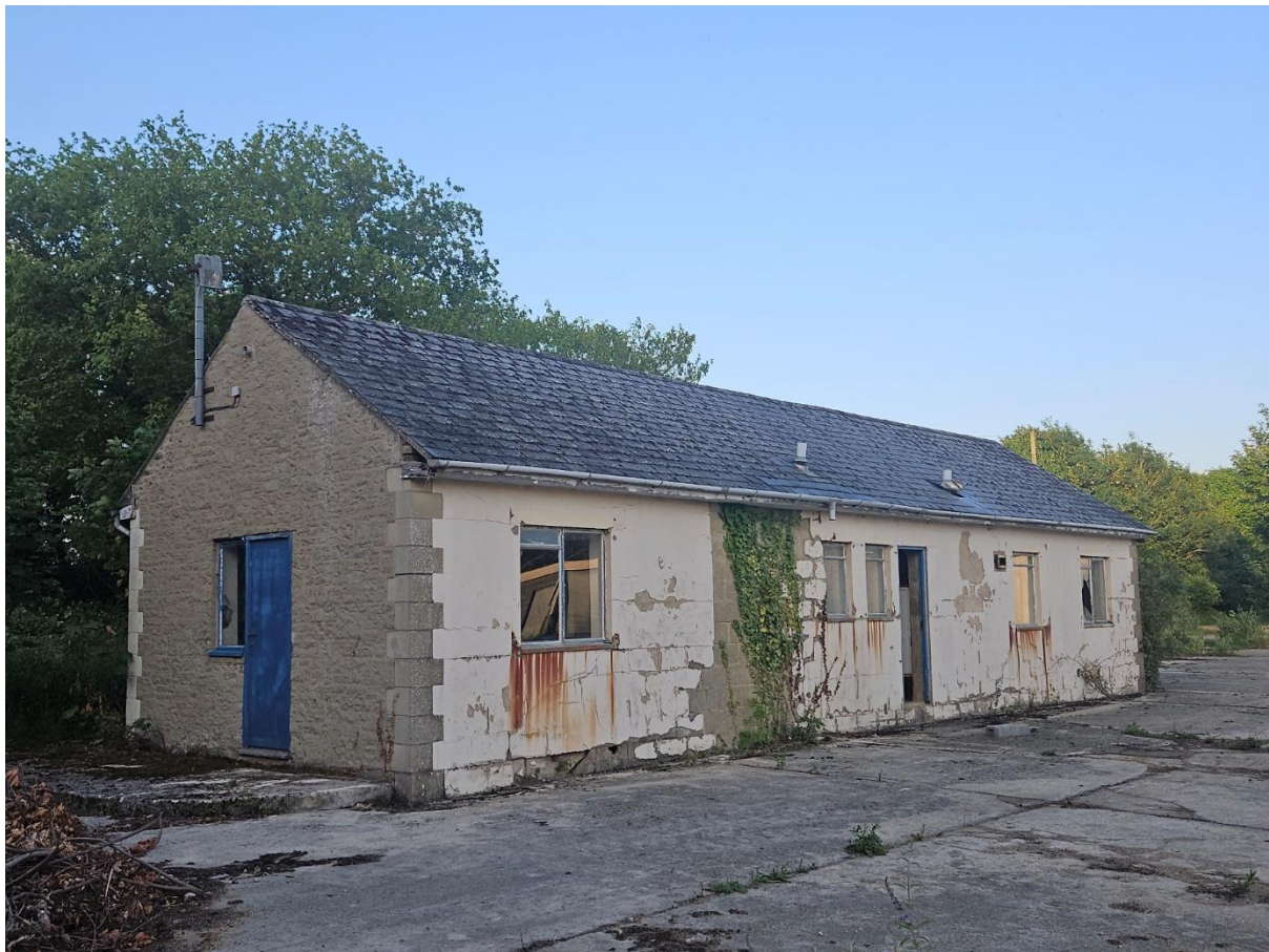
Photograph 2: showing a view of the target building (facing north-east)
