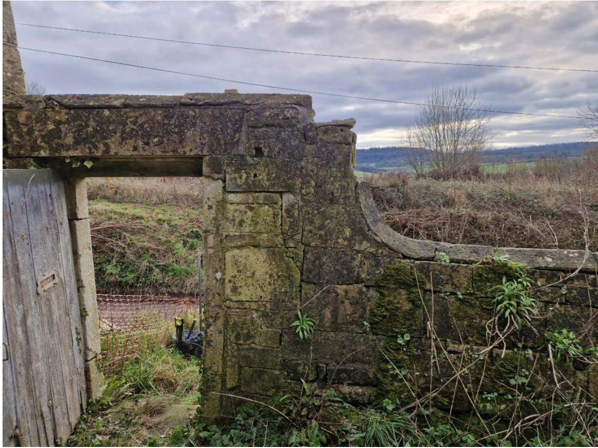
Photo 5: The subsidiary rear gated access and its moulded, ramped stone coping, with the boundary wall continuing beyond.
