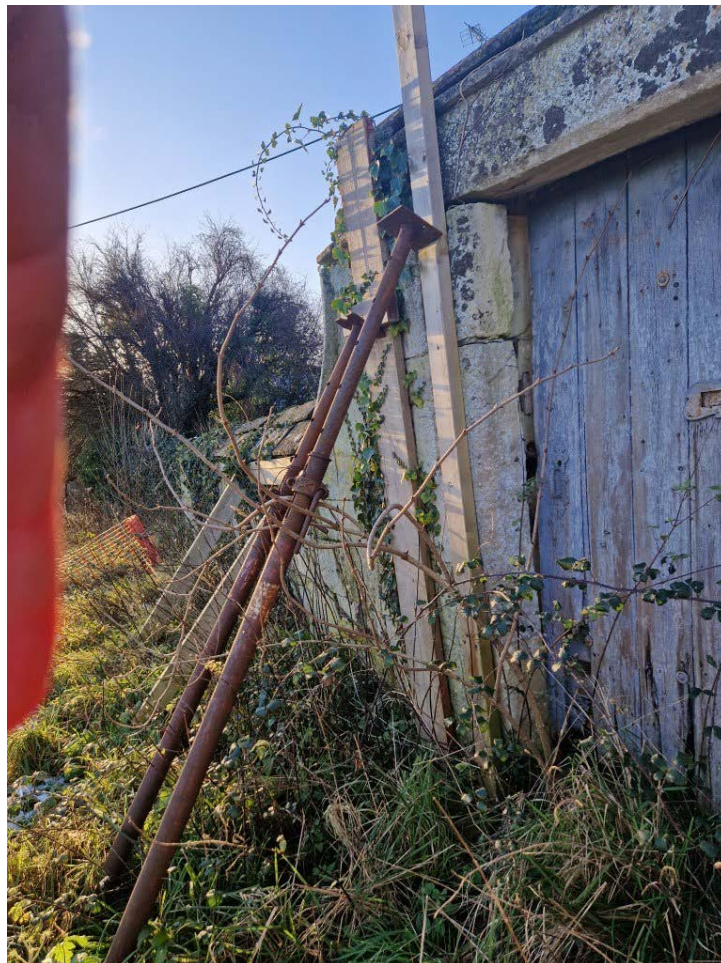
Photo 2: Detail of the temporary timber and steel raking shores installed against the gate pier and adjoining wall as an interim safety measure.
