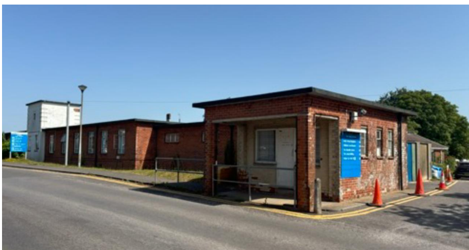
Figure 2.3 Building 15 (central tower block shown to the left and the access road to the existing car park shown to the right of the photo)
