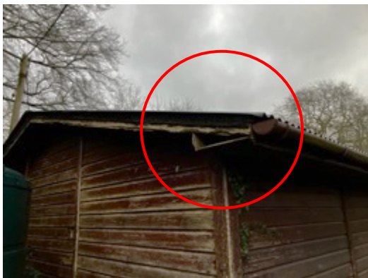
Photograph 23: Single PRF on the Garage
