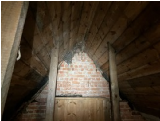
Photograph 19: Void 3 looking eastward
