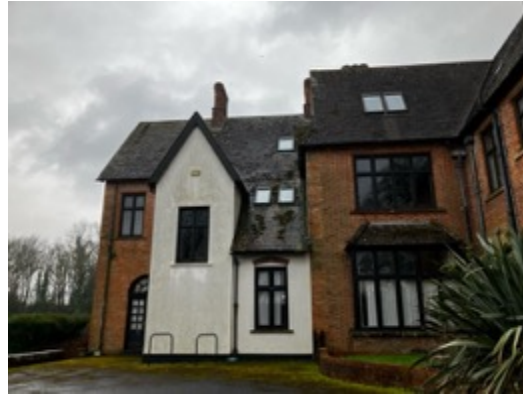
Photograph 14: Northeast elevation of Eastleigh Court
