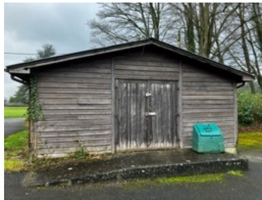
Photograph 22: Eastern elevation of the Garage
