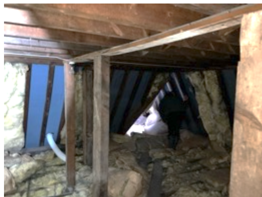
Photograph 18: Void 2 looking northward
