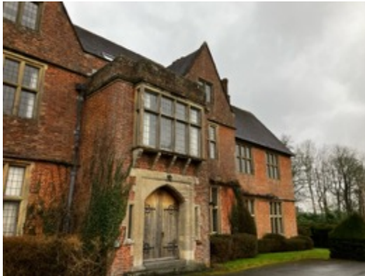
Photograph 13: Southern elevation Eastleigh Court
