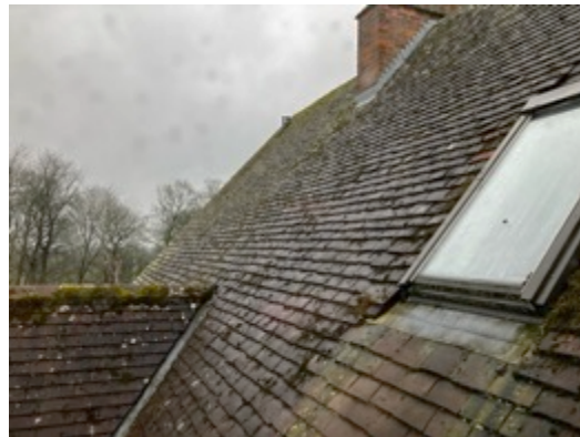
Photograph 16: View of roof with PRFs
