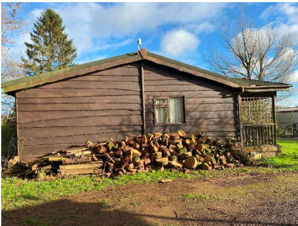
Photograph 17. B2 – western elevation
