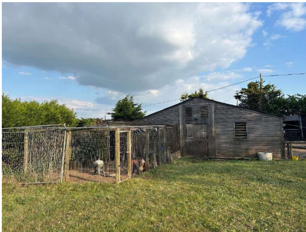
Photograph 29. B6 – northern elevation
