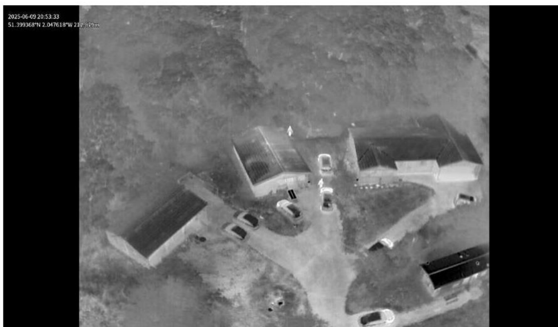
Figure 21: Survey 2: Position 8: Start: Mungo Nash, DJI MAVIC 3E/3T drone
