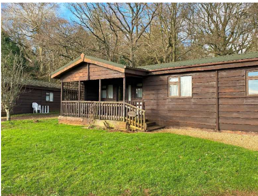
Photograph 14. B2 – south-west corner
