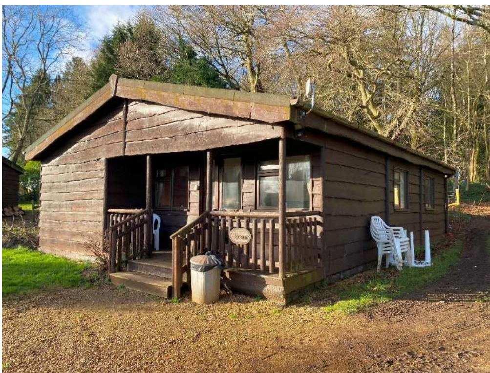
Photograph 18. B3 – from the south-eastern corner
