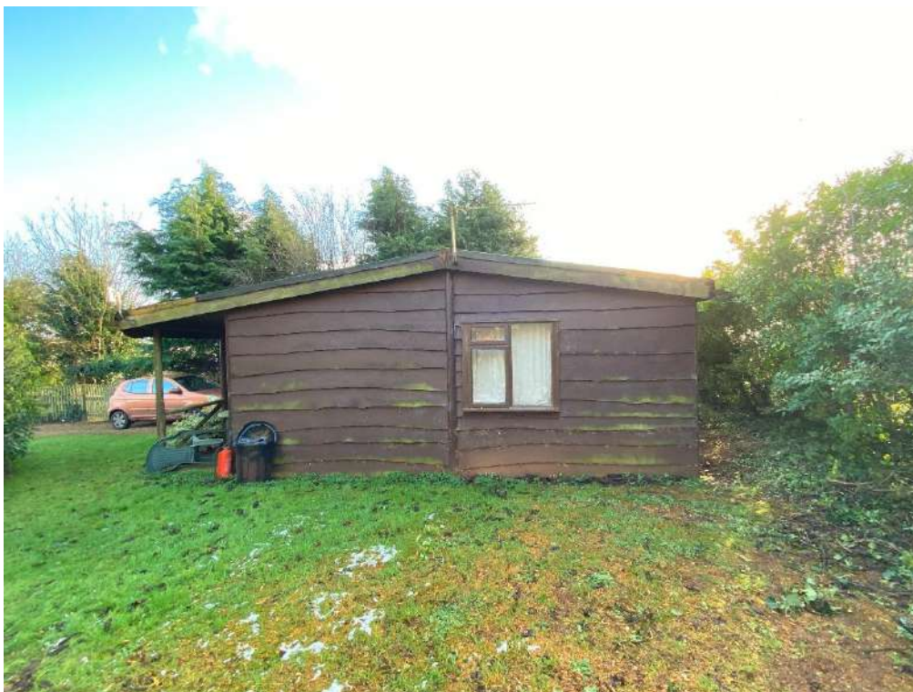
Photograph 23. B5 – northern elevation
