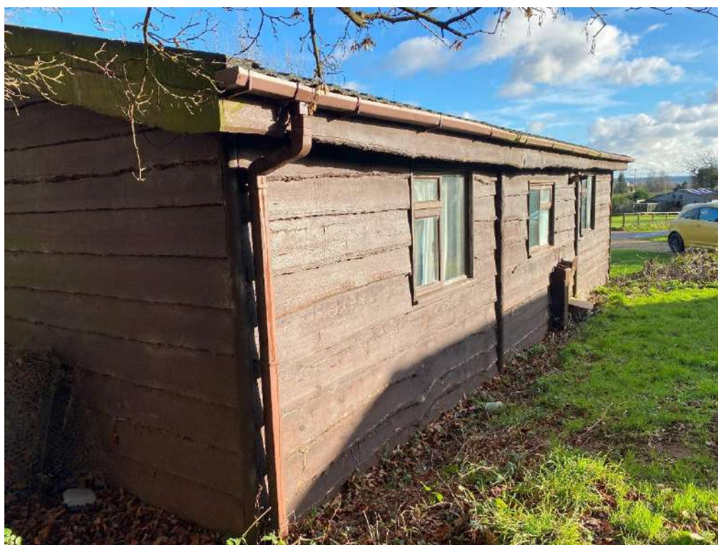
Photograph 20. B3 – western elevation
