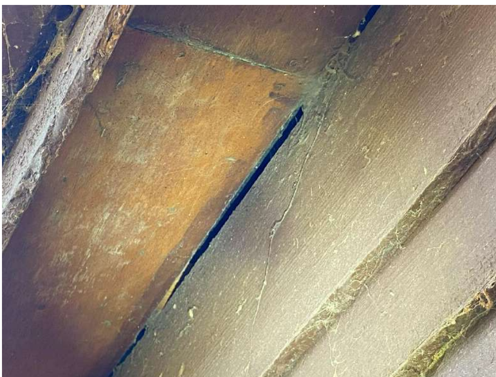
Photograph 40. PRF on the southern elevation of B2
