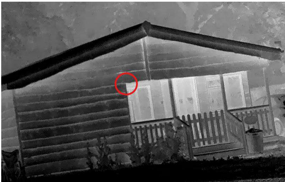
Figure 4: R1: common pipistrelle roost access point
