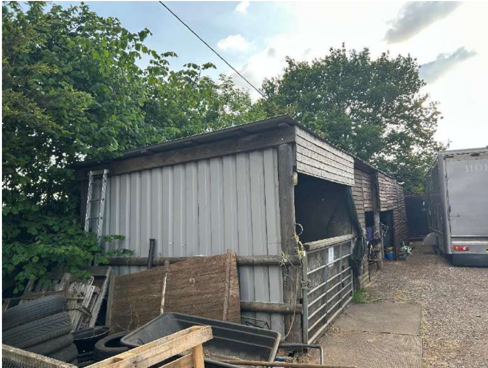
Photograph 31. B7 – northern and western elevations
