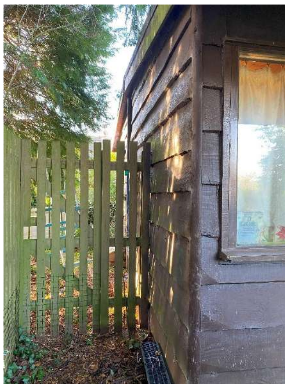
Photograph 25. B5 – southern elevation
