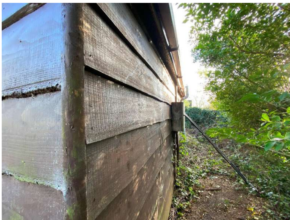
Photograph 26. B5 – western elevation
