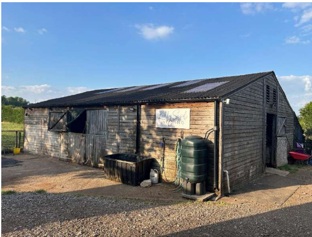
Photograph 27. B6 – western and southern elevations
