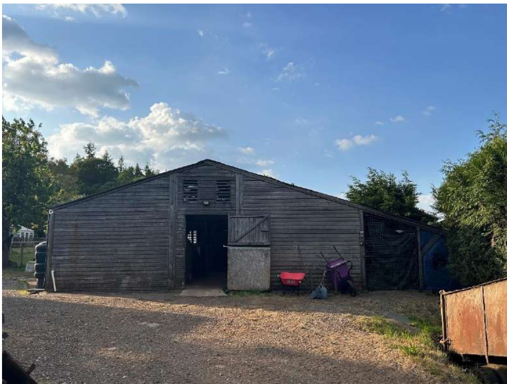
Photograph 11. Curtilage of unsealed surface around the stable block
