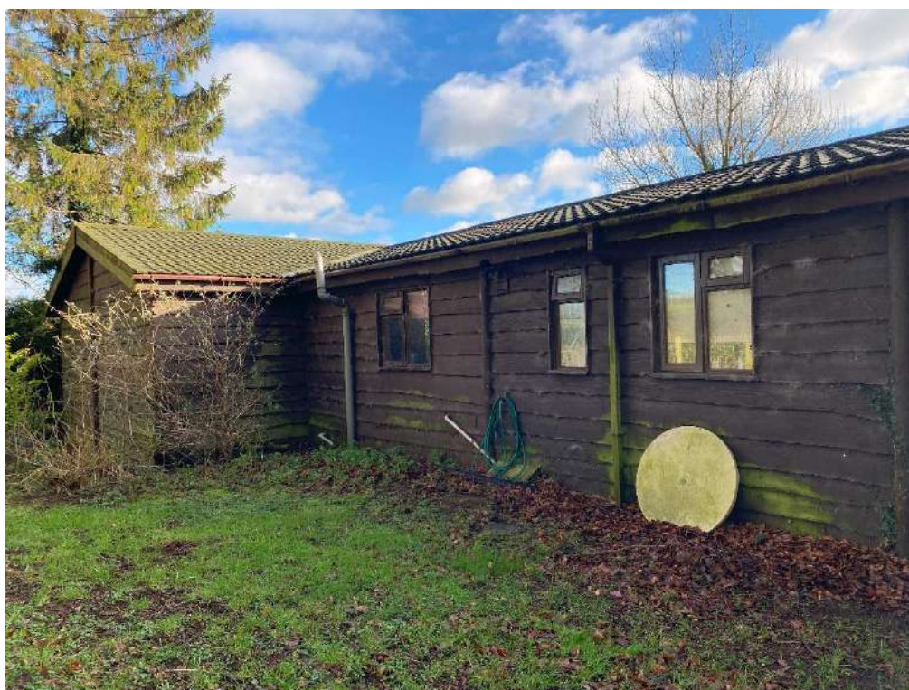
Photograph 16. B2 – northern elevation
