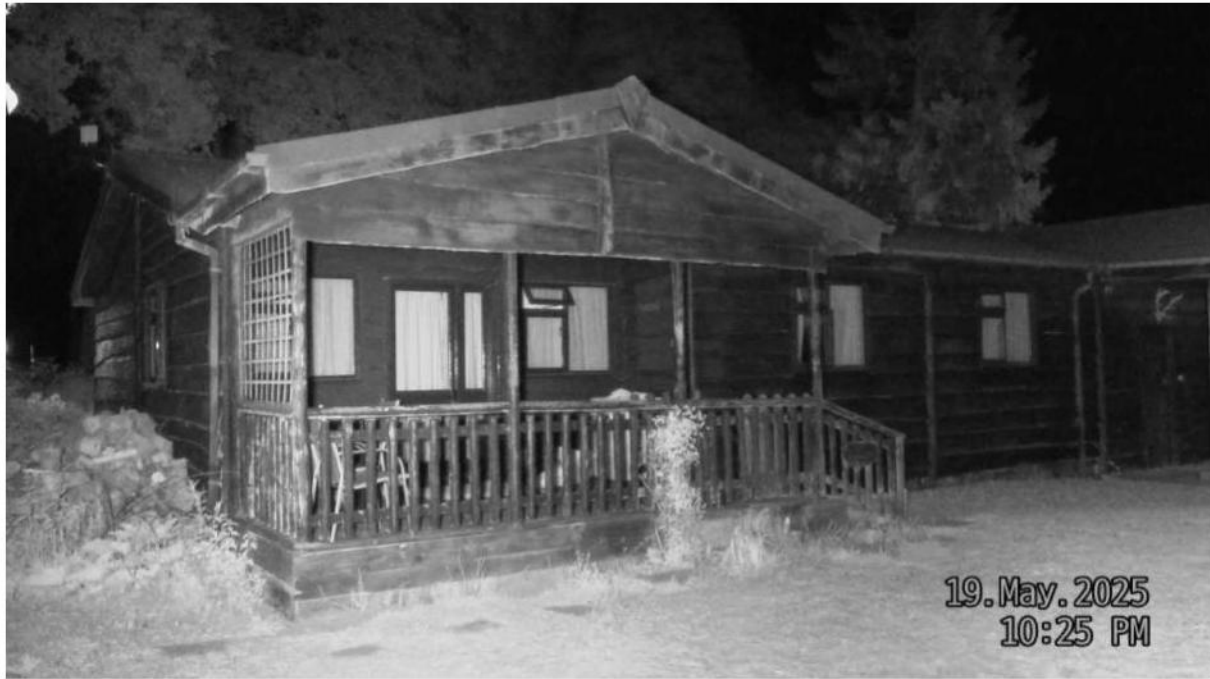
Figure 10: Survey 1: Position 2: End: Standalone, Canon XA60
