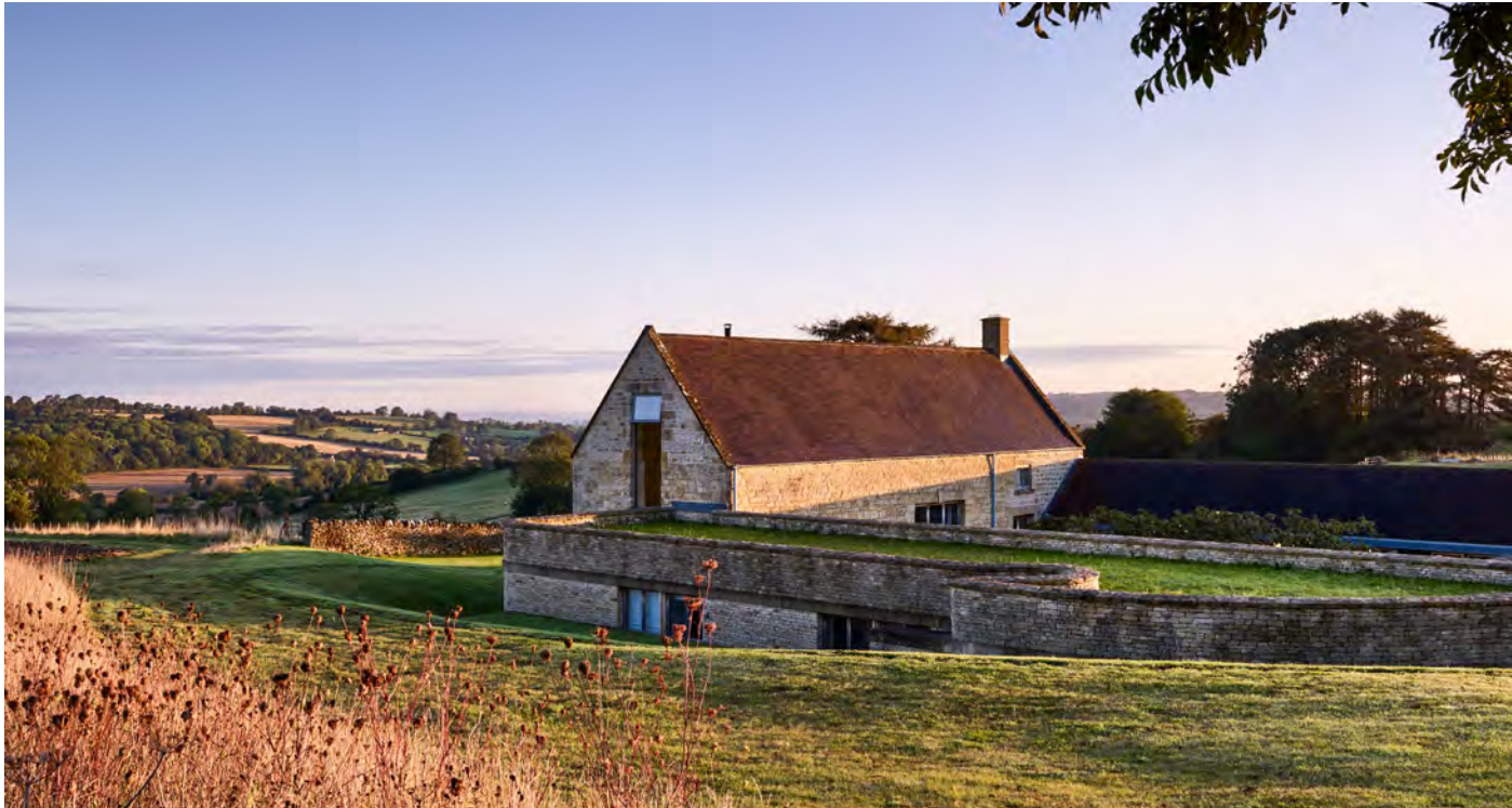
Cotswold Barn Conversion Chipping Campden, Gloucestershire
