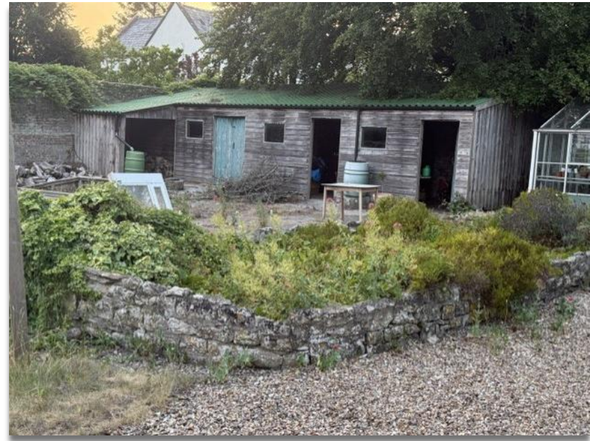
Figure 5. Existing timber sheds to north boundary wall. Timber log store to west boundary wall. Proposed location of garage to the south of this range, to west boundary wall.
