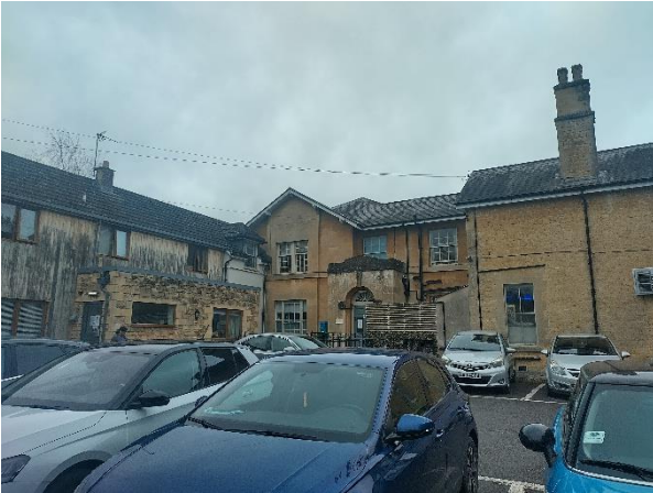
Photograph 1: View of the southern and eastern elevations, facing northwest.
