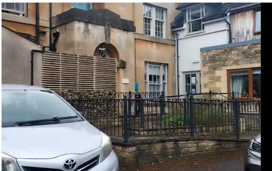
Photograph 3: Access ramp to be removed to facilitate the eastern extension.
