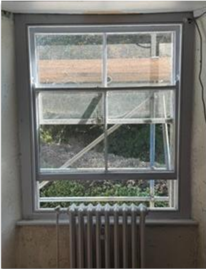
Figures 14 and 15. Modern replica sash windows (to be replaced).
