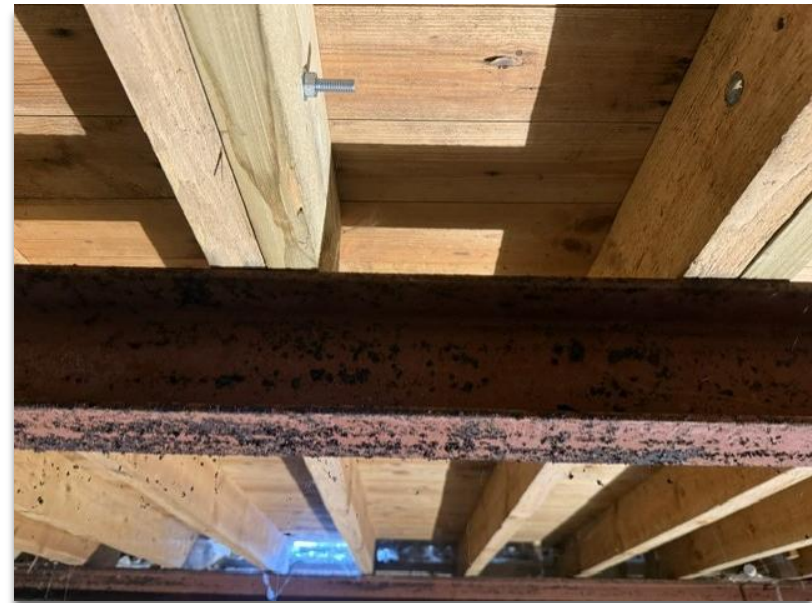
Figures 7 and 8. Cellar ceiling, comprising C20 timbers supporting the C20 proposed kitchen floor (pine) above.
