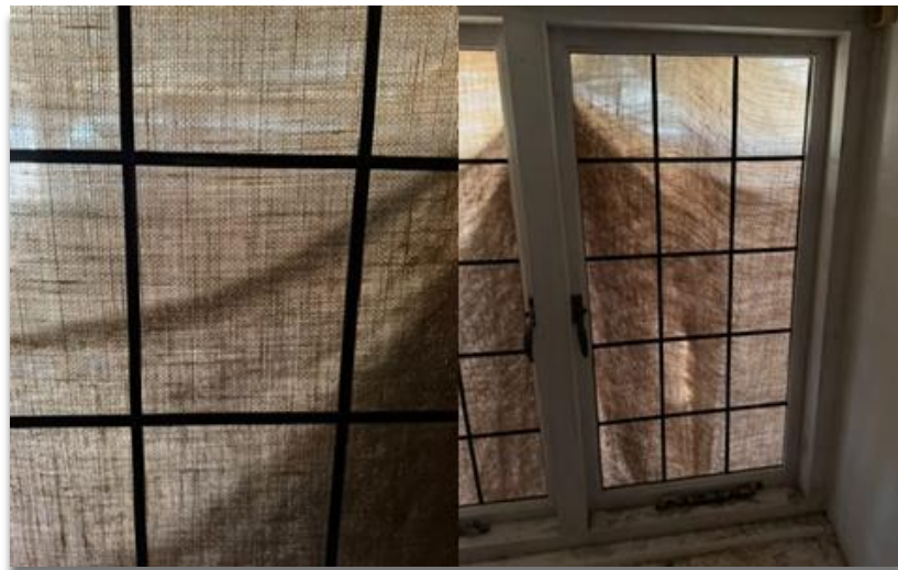
Figures 9 and 10. First floor bathroom window (c. 2023). Stick on faux lead. Proposed to be replaced with existing kitchen window (south).
