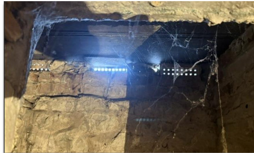
Figure 3. Cellar lightwell looking up towards area outside existing east door (proposed kitchen).
