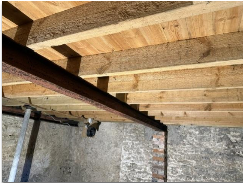
Figures 7 and 8. Cellar ceiling, comprising C20 timbers supporting the C20 proposed kitchen floor (pine) above.
