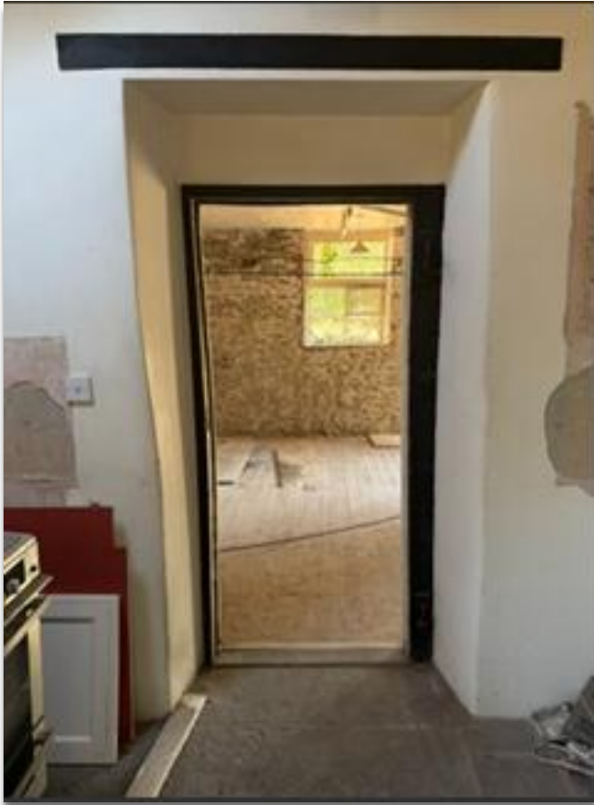
Figure 5. Looking north towards proposed kitchen/dining room door opening.
