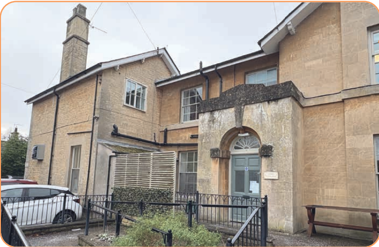
The former main entrance, now a service entrance beside the parking area, is well placed and of suitable historic character to resume its role as the building's principal entrance.
