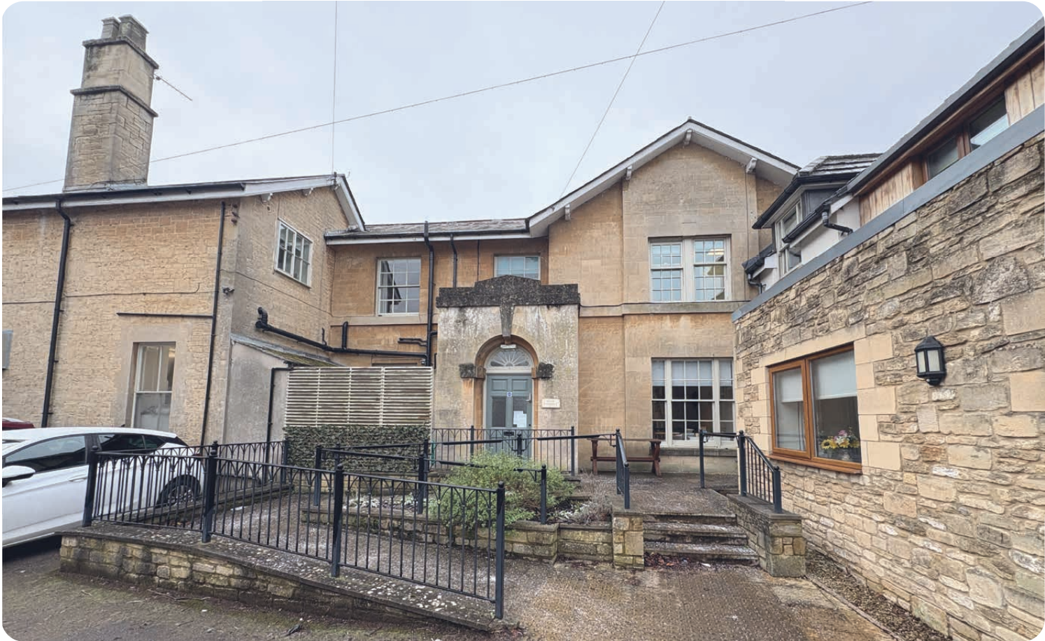
1. Existing Front Elevation - Not currently used as main entrance
