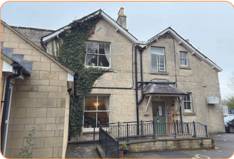
Existing main entrance into the building is currently discretely located out of view from the main car-park disorientating visitors.
