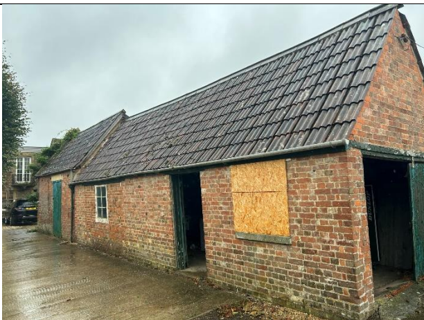
Photograph 3: Building 6 – Estate Office N gable and E elevation.
