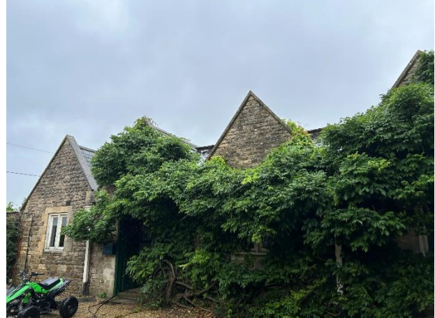
Photograph 2: Buildings 5,7 and 6 southern elevation.
