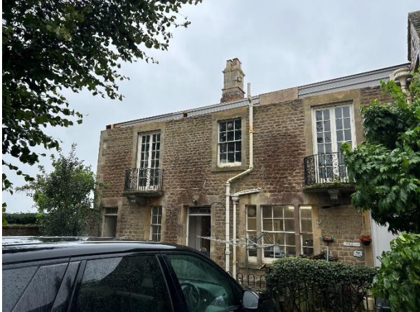
Photograph 1: Building 2 northern elevation.
