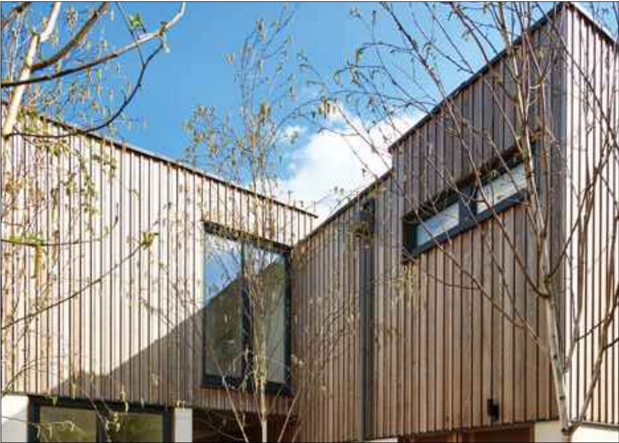
Timber Cladding - Vastern Brimstone Ash Square Edge VHL 4 vertical cladding 20mm thick, 140mm wide
