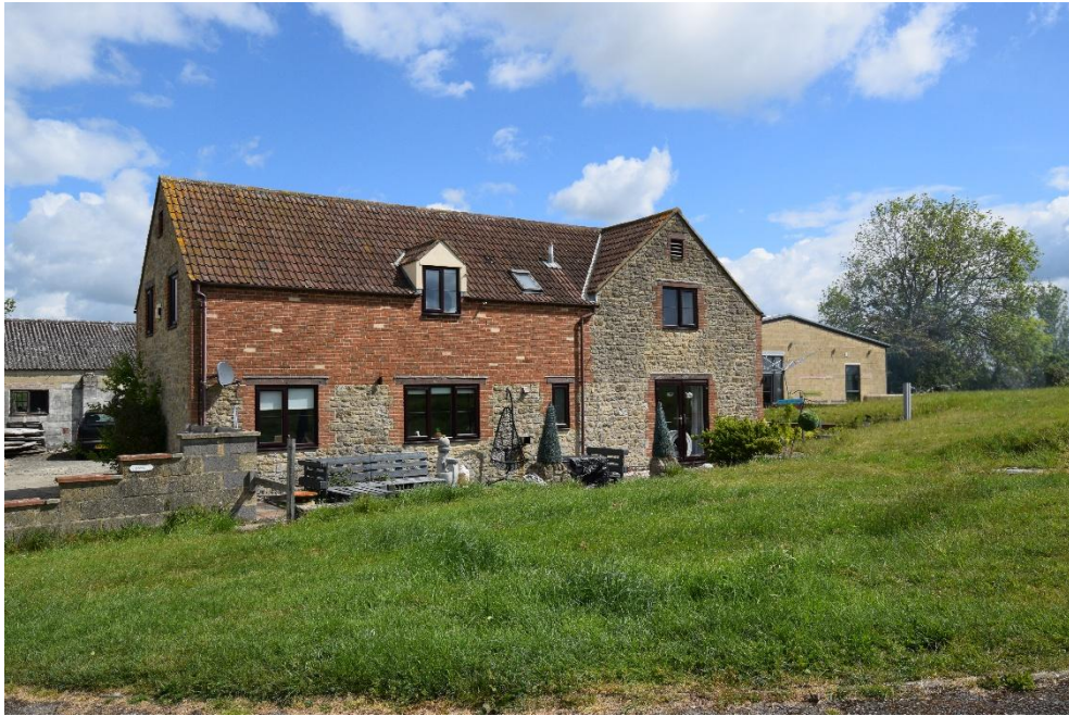
The Cottage – Front (South Elevation)
