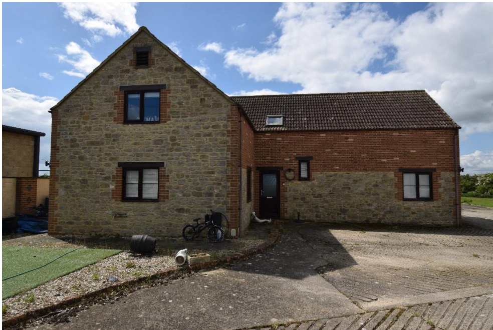
The Cottage – Rear (North Elevation)
