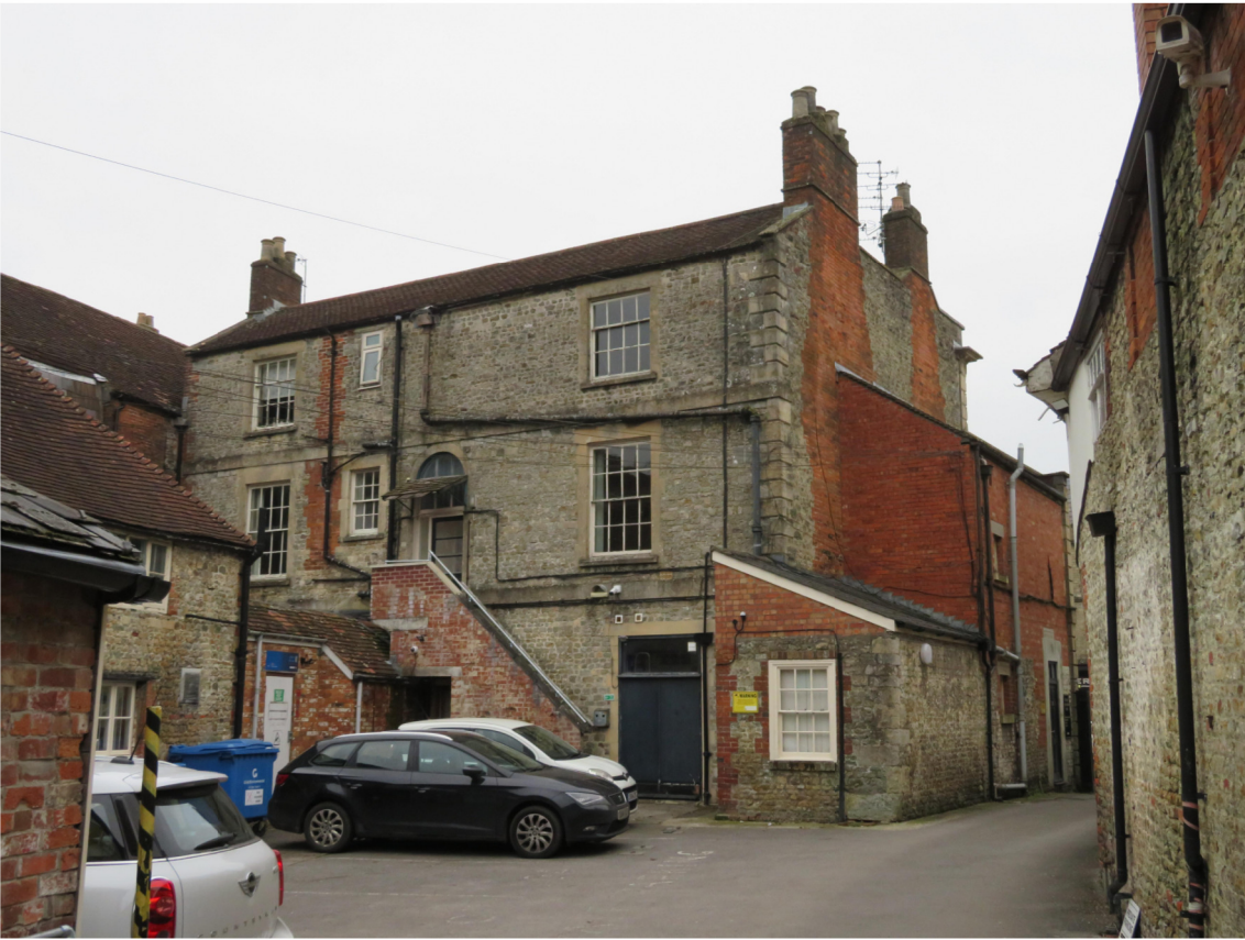
PHOTO OF EXISTING BUILDING REAR
