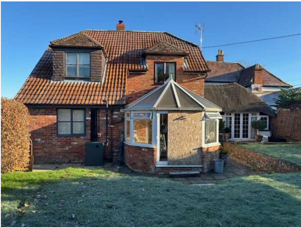
View of the south-west elevation of Dairy Cottage.
