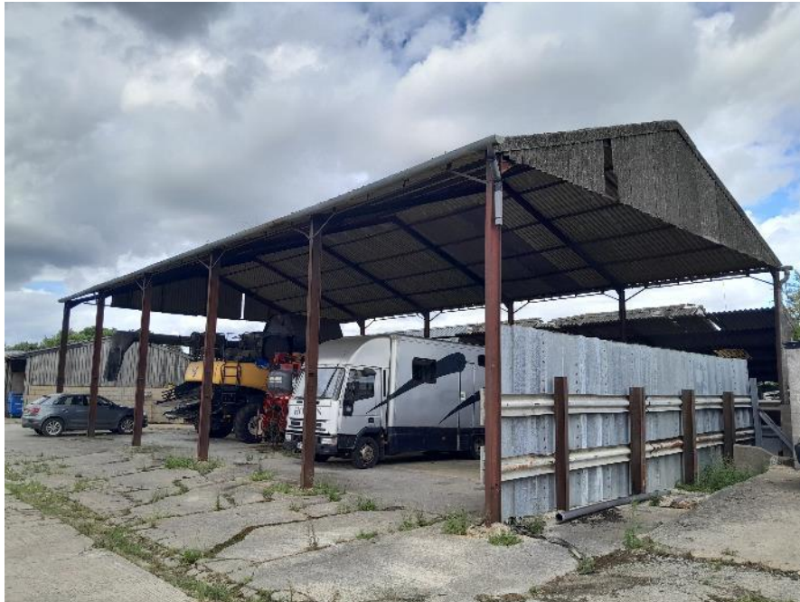
Photo 16. Western and southern elevations of B7
