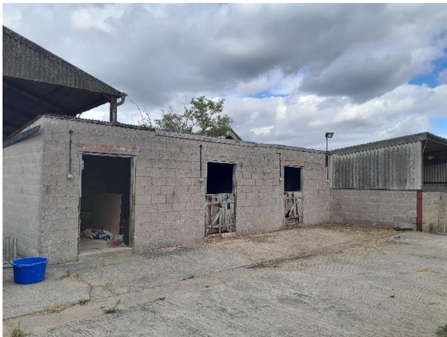
Photo 17. Southern elevation of B8
