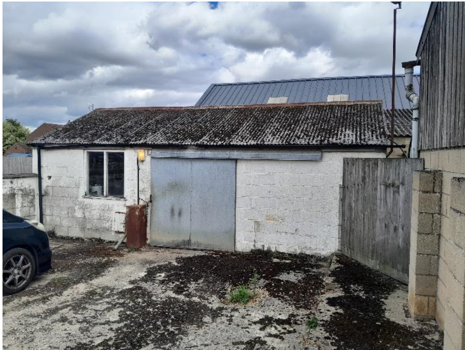
Photo 4. Western elevation of B2
