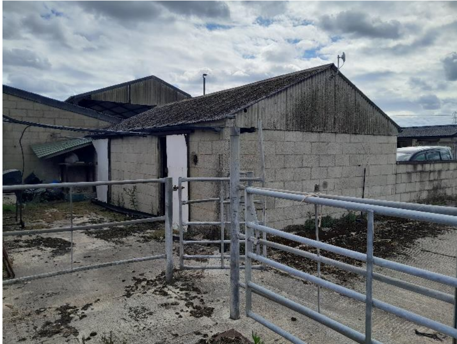
Photo 5. Northern and eastern elevation of B2
