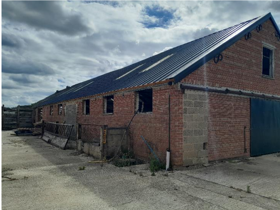
Photo 9. Northern and eastern elevations of B4
