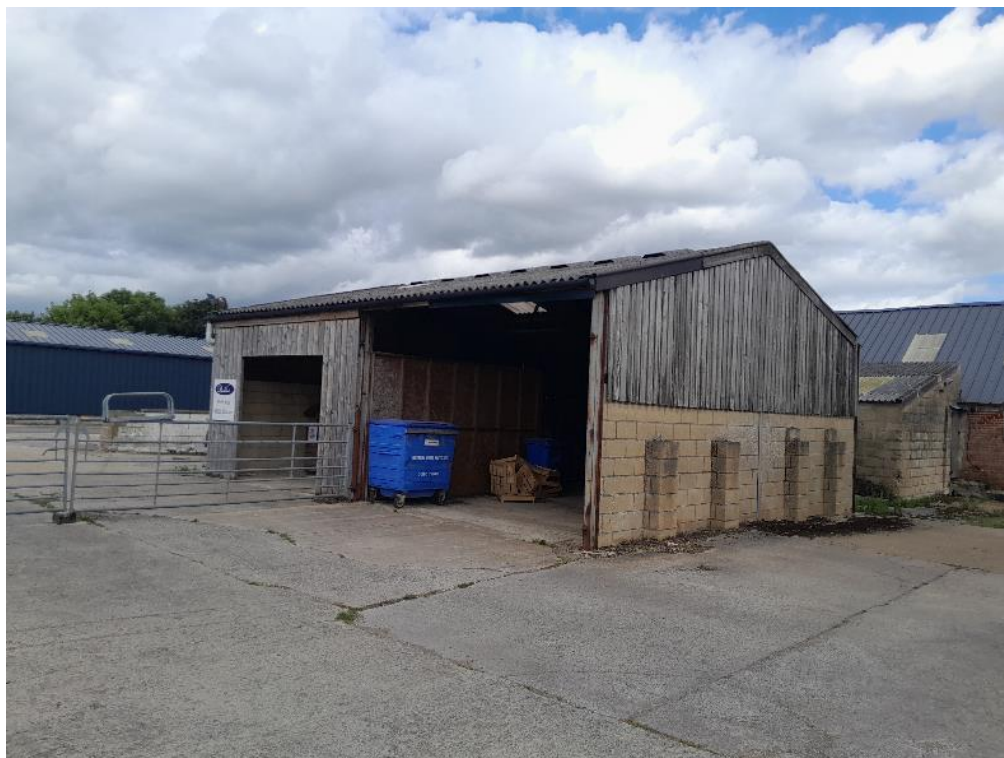
Photo 1. Southern and eastern elevation of B1
