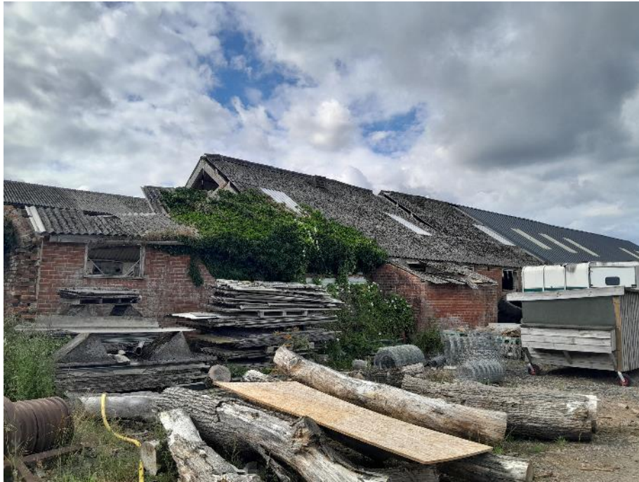
Photo 12. Eastern elevation of B5 and B9
