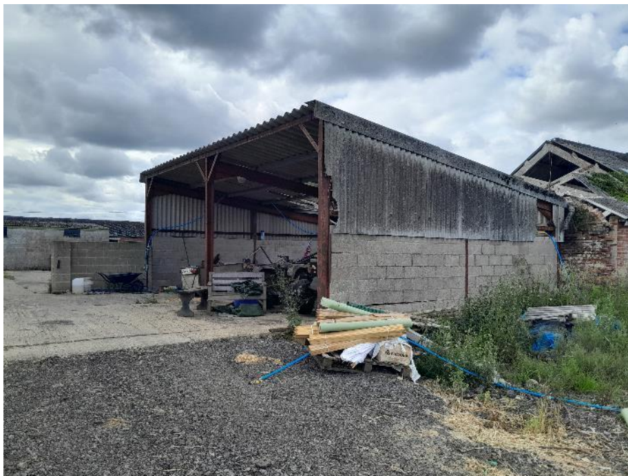
Photo 19. Southern and eastern elevations of B9
