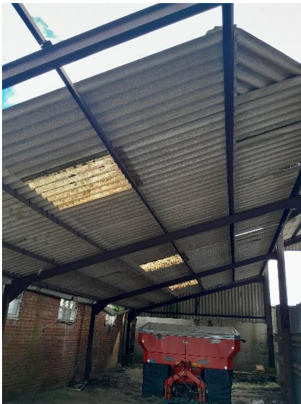
Photo 15. Roof structure of B6
