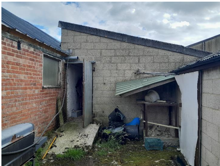
Photo 7. Northern elevation of B3
