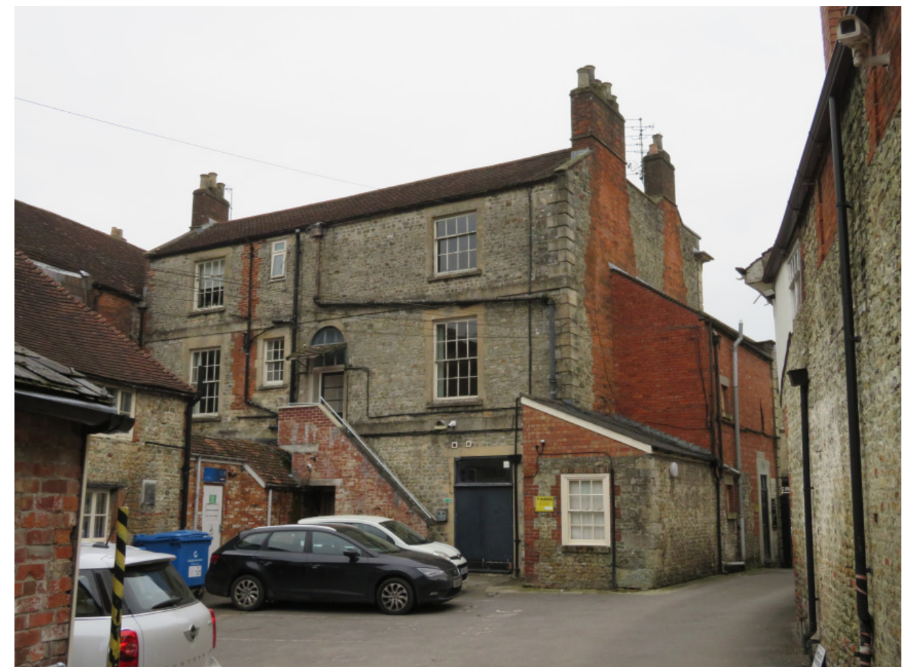
FIG.6 Looking at rear of building
