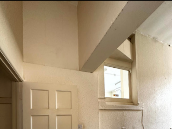
FIG.16 Side Stairwell internal window
