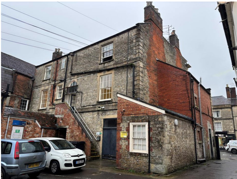
Fig.4 Back of the building; external steps to the first floor
