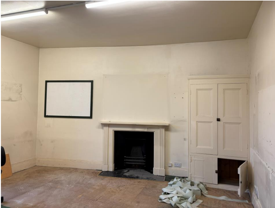
Fig.7 Room 1 (left-hand rear) – simple timber fireplace and historic built-in cupboard
