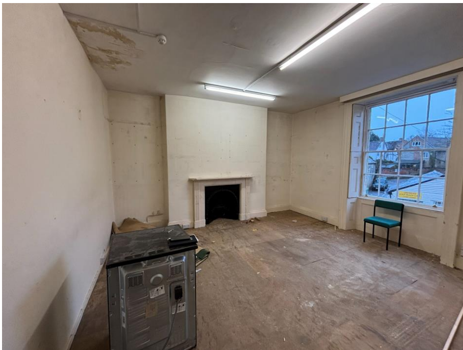
Fig.10 Room 6 (right-hand rear) - note general plainness, lack of cornice etc
