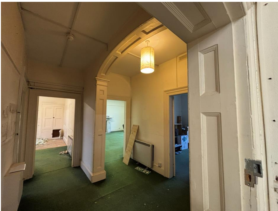
Fig.6 Arched opening within the landing
