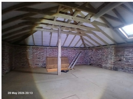
Loft void of B2 taken from the northwestern corner.
