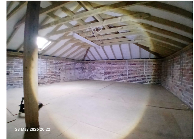
Figure 1a: Loft void of B2 taken from the northeastern corner.
