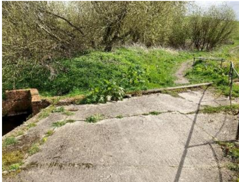
Figure 7: Concrete slab over dam headwall
