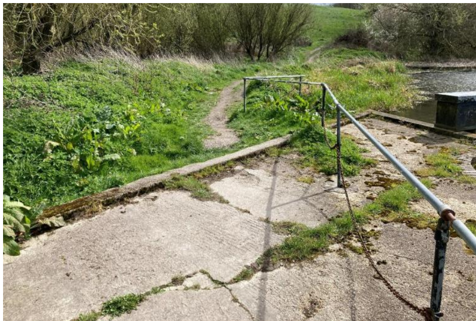
Figure 8: Footpath on earth embankment to be topped up to make slab
