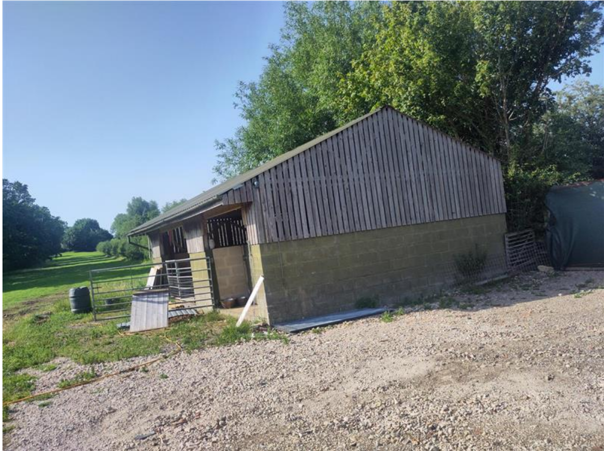
Photograph 1: an exterior view of the barn (facing north-west)
