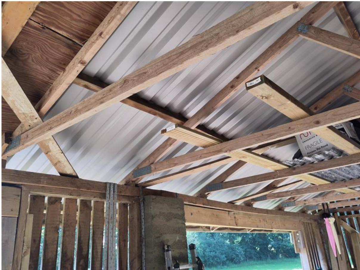
Photograph 4: showing a view of the internal roof of the barn (facing north-west)
