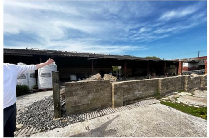
Below - Barn 2- southeast elevation facing into the yard
