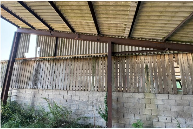
Barn B2 junction with B1.
