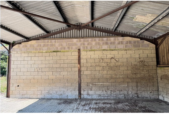
North gable end of Barn B1
