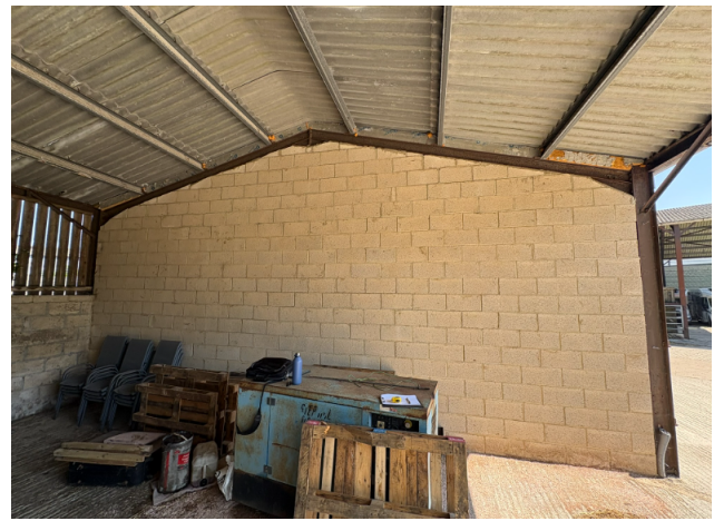
View of storage area within Barn B1 (not accessible)
