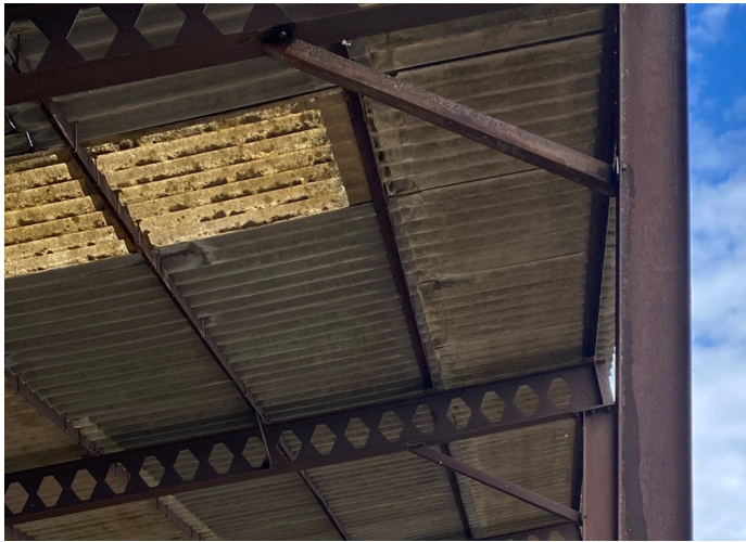
Barn B2 knee-brace detail between stanchion and castellated roof beams
