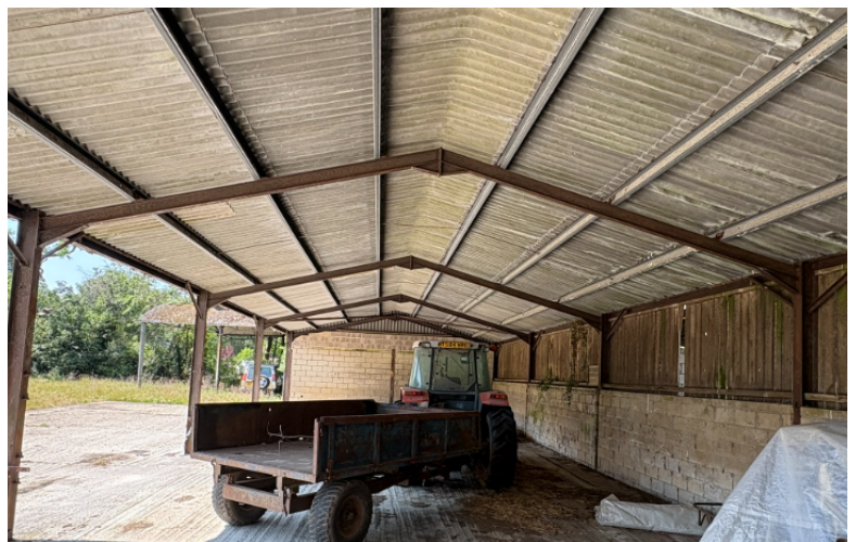
Typical portal frame view (Barn B1)
