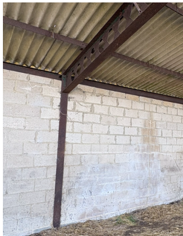
Lower eaves detail to Barn B2
