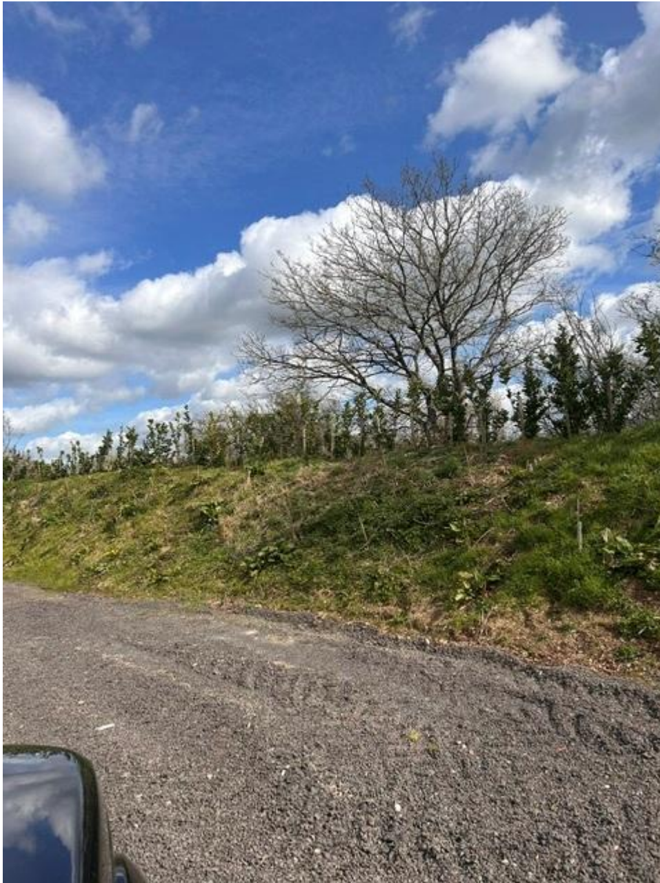
Figure 4 Photo of earth bund, and demonstrating planting of trees into earth-mound bund for further concealment of the site from A350 view
