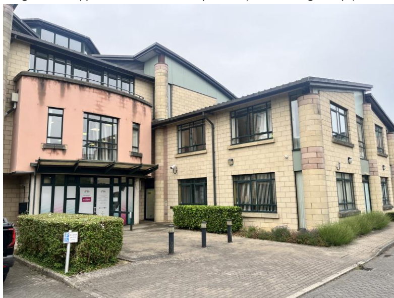
Image 2 – the application site building – Block A
