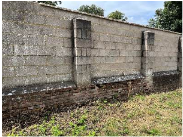
Figure 22 – example of one of the historic brick walls (left) / Figure 23 - example of one of the modern blockwork walls (right)
