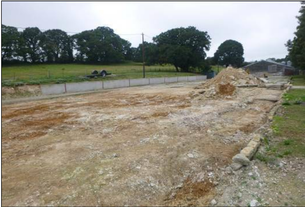
Photograph 9 Showing the southern section of the concrete base where concrete removal has begun
