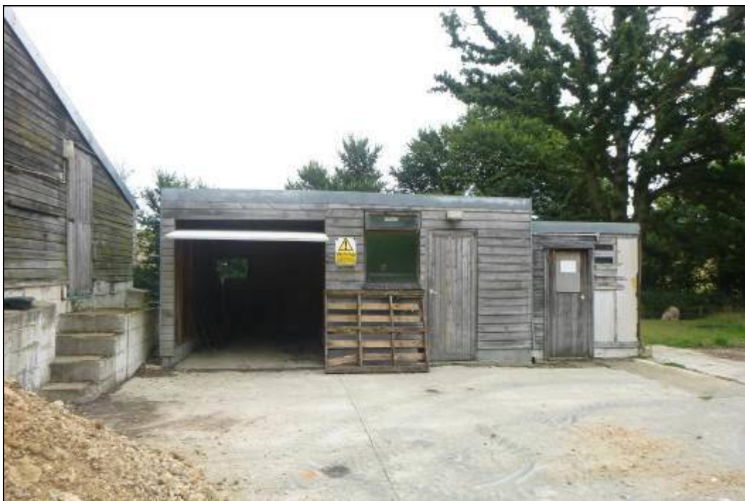
Photograph 6 Showing the courtyard and stable to the south of the existing poultry shed
