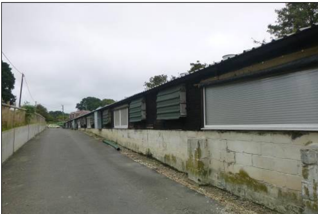
Photograph 4 Showing the tarmac section to the west of the existing poultry shed
