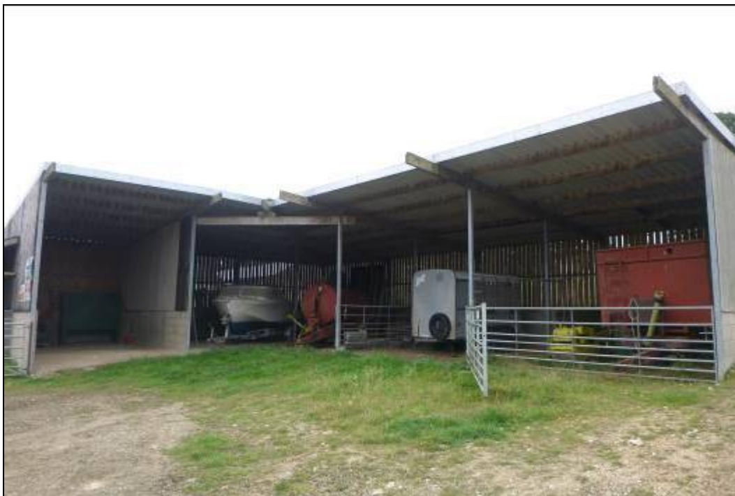
Photograph 10 Showing the open fronted barn in the southwestern corner of the site
