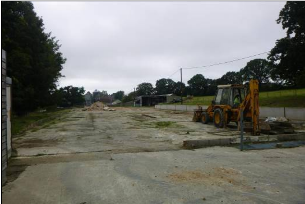
Photograph 7 Showing the concrete base of the demolished poultry shed from the northern end
