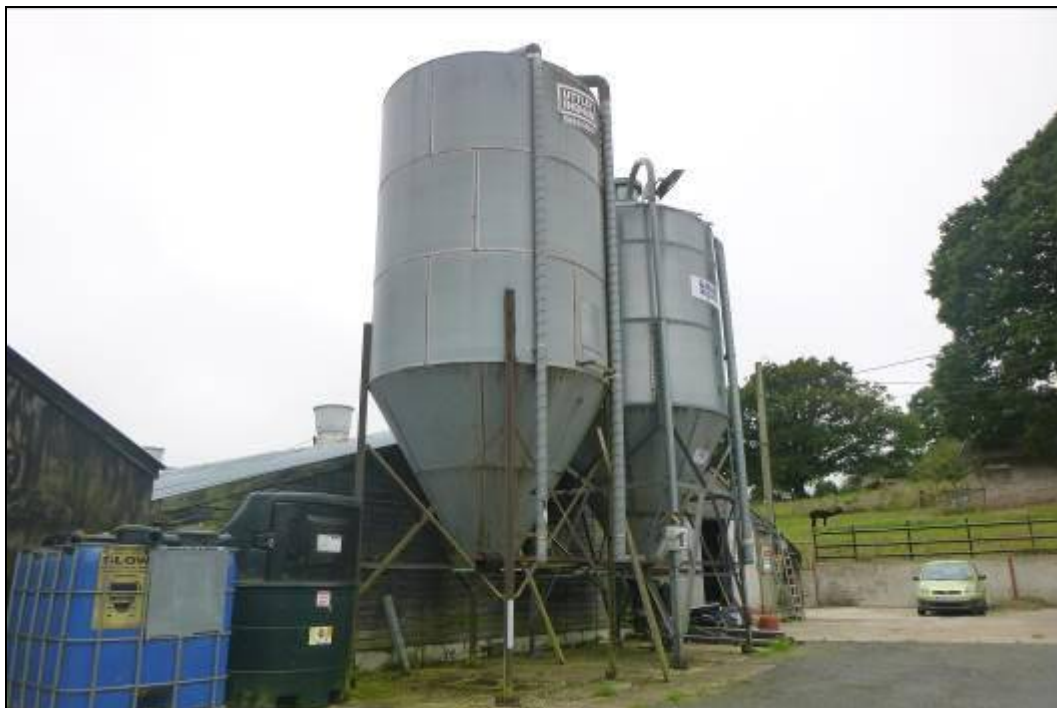
Photograph 2 Showing the concrete parking area with the grain silos, oil tank and vehicle disinfectant outside the northern end of the existing poultry shed
