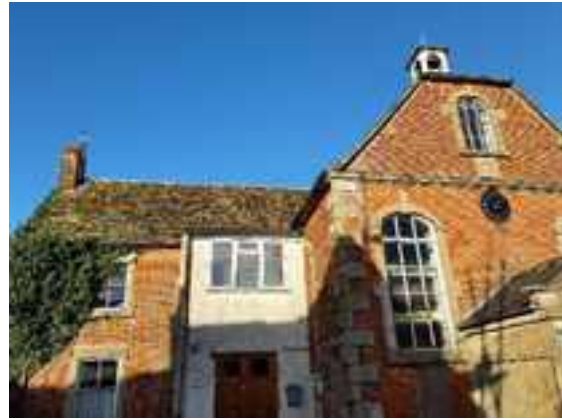
Figure 40: A view facing north-east of the main residential dwelling. The roof space on the left side is the “east-west” loft void
