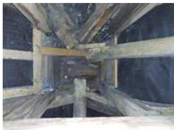
Figure 44: A view facing south from within the northern entrance of the north-south loft void
