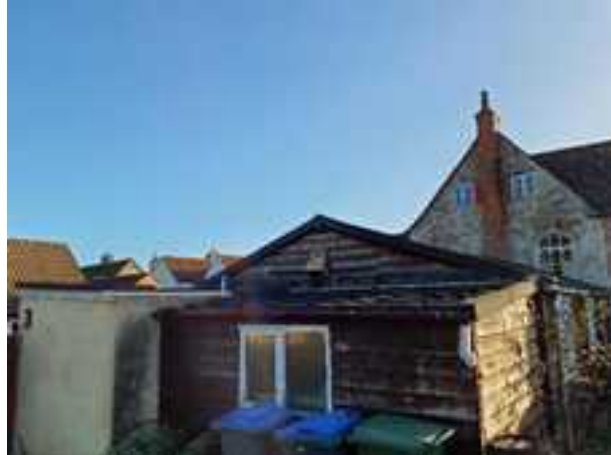
Figure 34: The east and north elevation of the main dwelling
