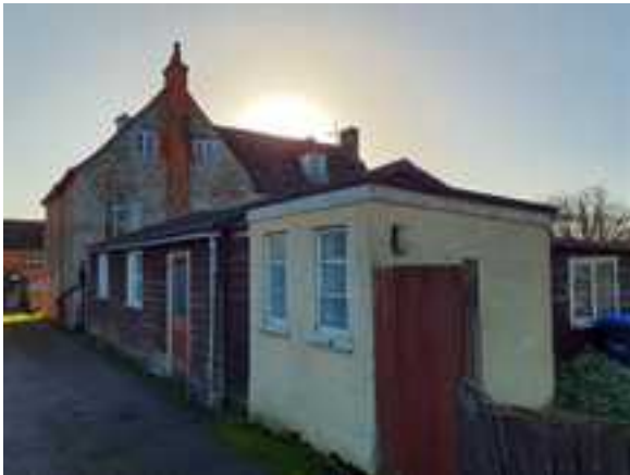
Figure 35: The south elevation of the main residential dwelling's chapel section as seen from the access path
