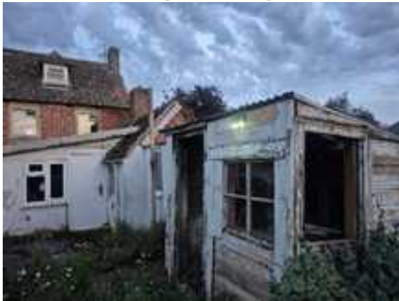
Figure 71: A light fitting on the east side of the shed with a high lux fitting
