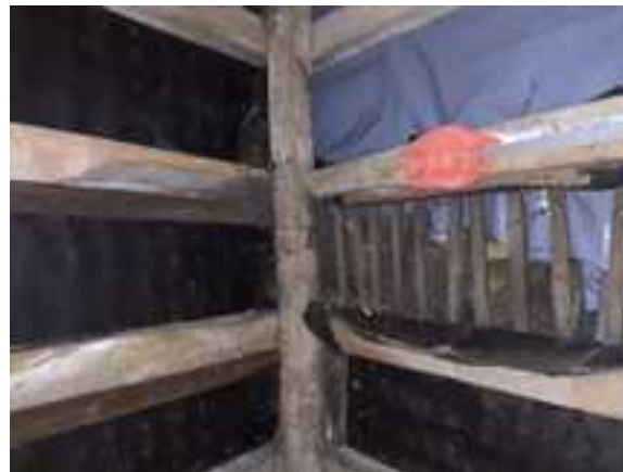
Figure 46: A view directly up from the northern entrance of the north-south loft void showing the only visible area of exposed tile due to deterioration of the roofing membrane
