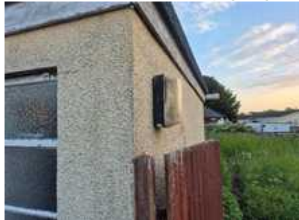
Figure 72: A light fitting on the west side of the dancehall which includes uplighting
