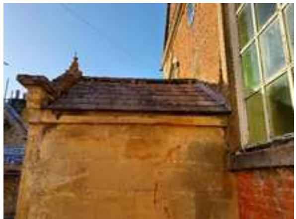
Figure 38: The south elevation of the main residential dwelling
