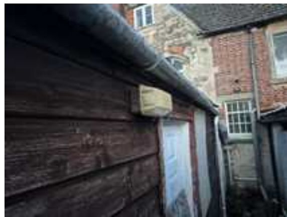
Figure 74: A light fitting on the west side of the dancehall which includes uplighting
