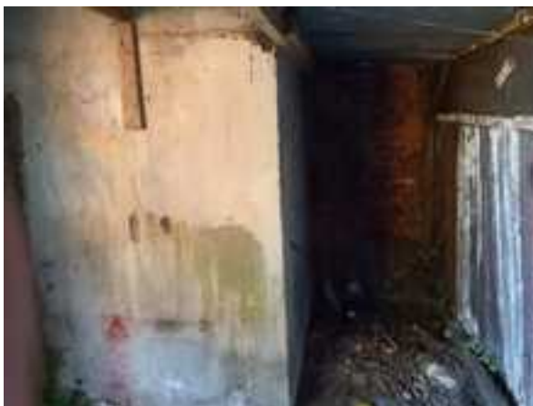
Figure 29: Inside the shed facing south to show the edge of the main dwelling's extension
