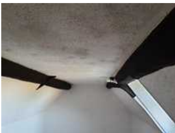
Figure 43: A view facing north from within the southern entrance of the north-south loft void
