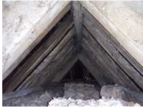
Figure 46: A view directly up from the northern entrance of the north-south loft void showing the only visible area of exposed tile due to deterioration of the roofing membrane
