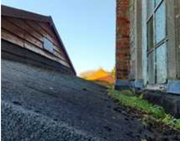
Figure 33: The east and north elevation of the dance hall as seen from the access road
