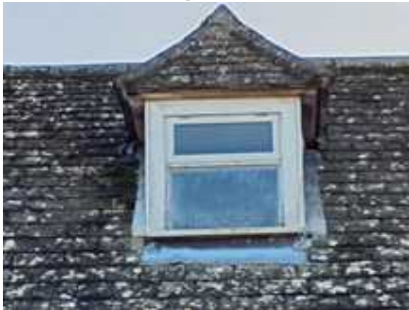
Figure 53: Raised flashing around the dormer window on the northern elevation of the main dwelling
