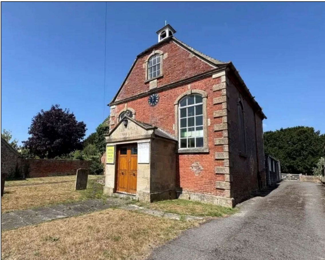
Photo 2 - Side Elevation and Driveway
