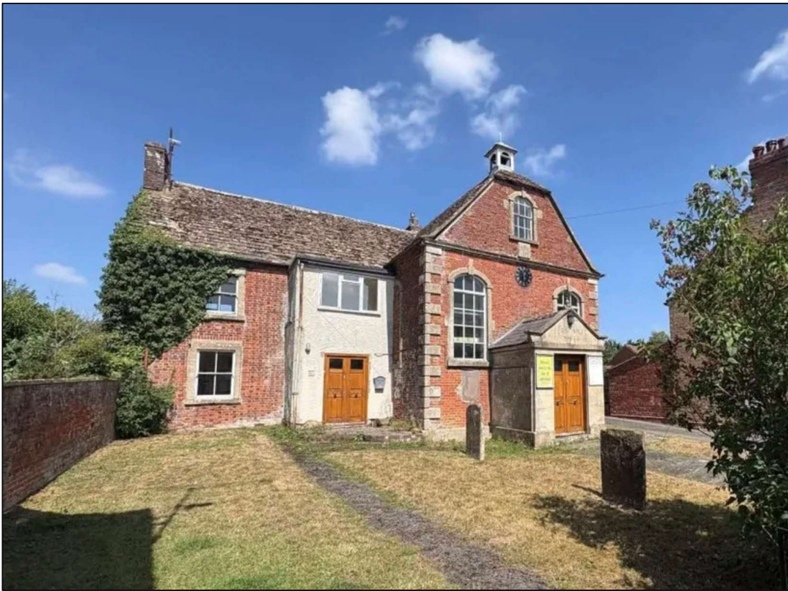
Photo 1 - Chapel and Manse - Front Elevation
