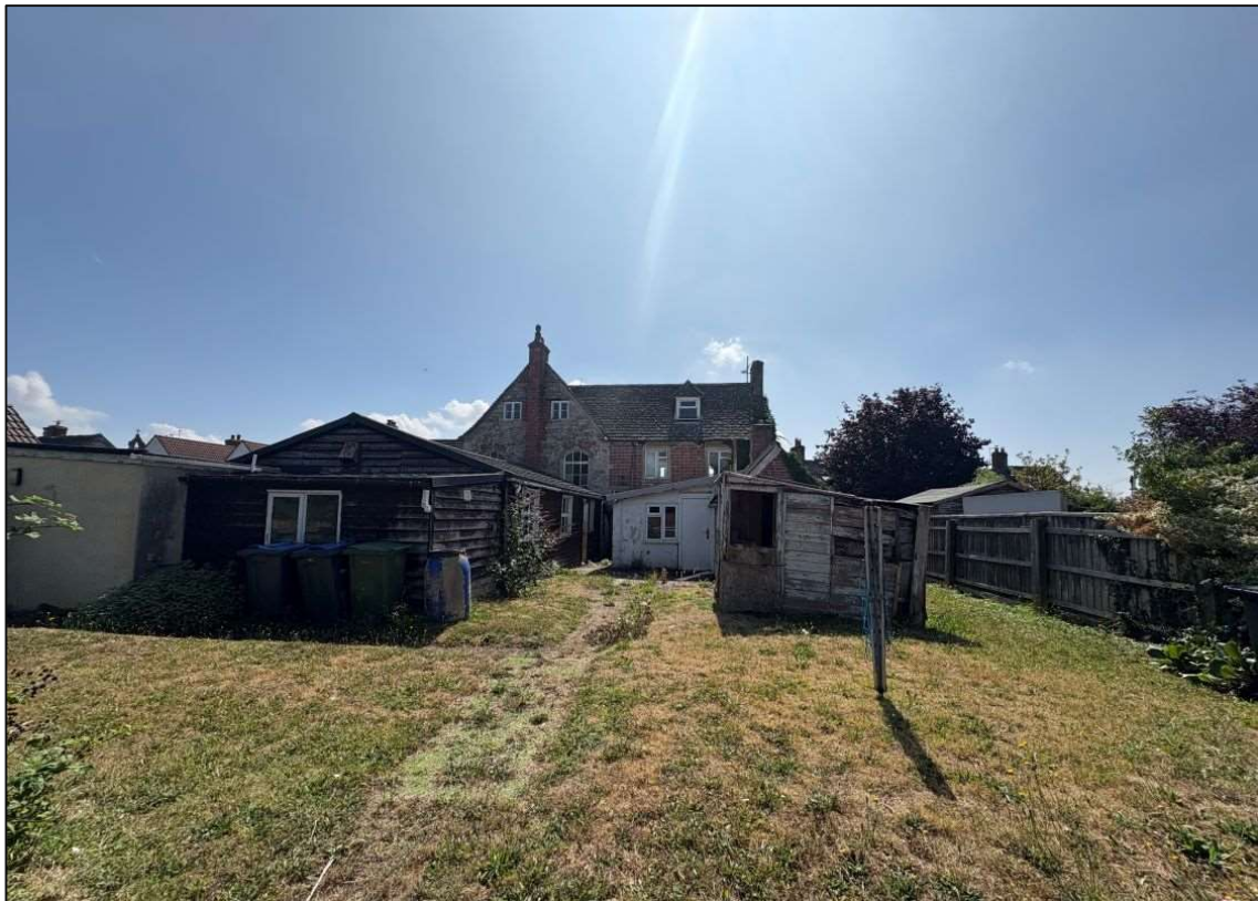
Photo 5 - Rear Elevation and Garden
