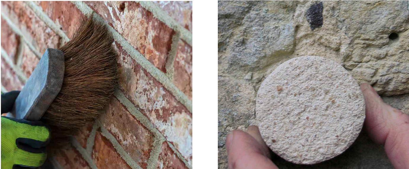
Image left: Brickwork to be reinstated and traditional lime pointing to be used extend the life of the brick. Image right: A lime mortar 'biscuit' to help colour match to existing pointing on site.
