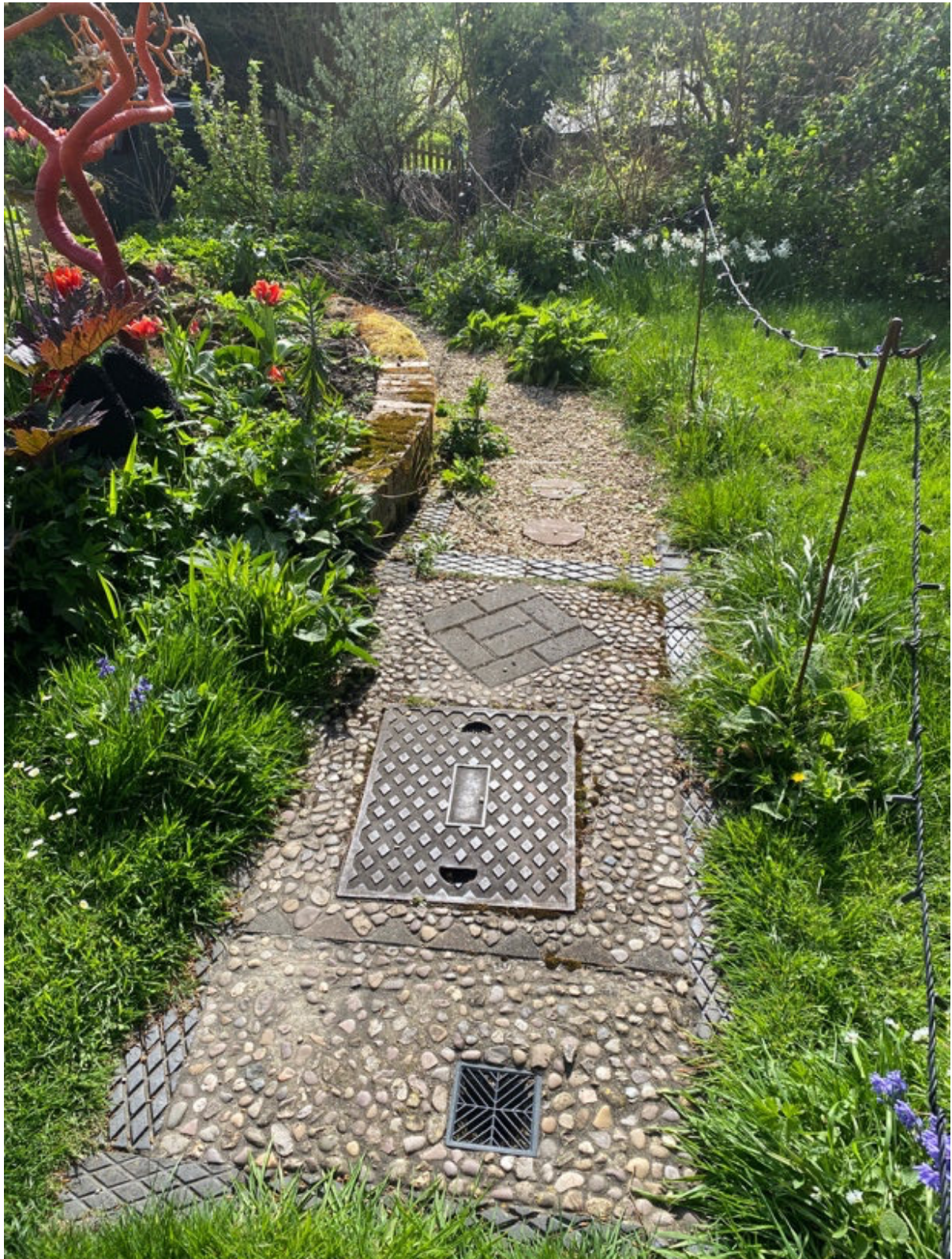
Photo to show manhole cover over existing double chamber septic tank at 45 High Street, Pewsey
