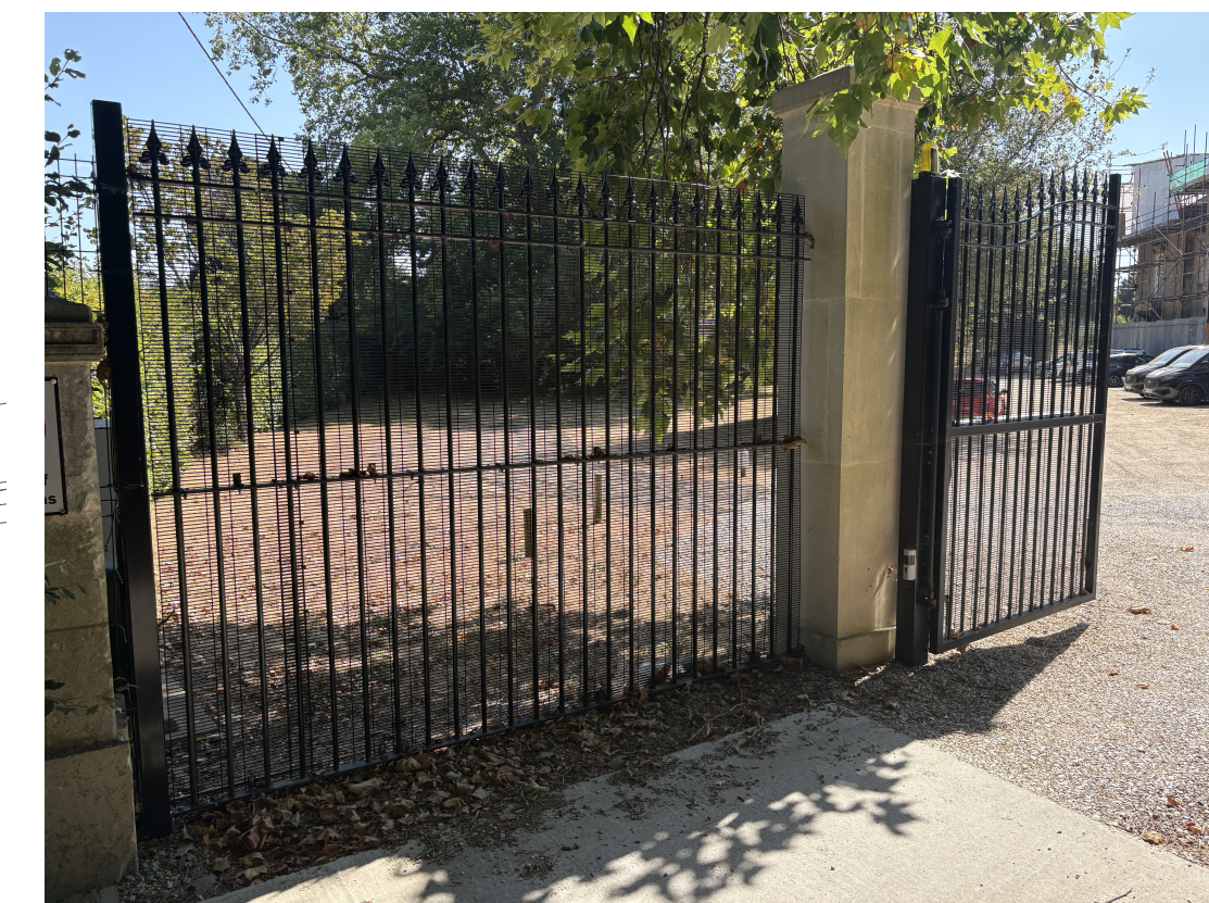
Photo from Notton School agreed and installed 5 years ago proposed fence
