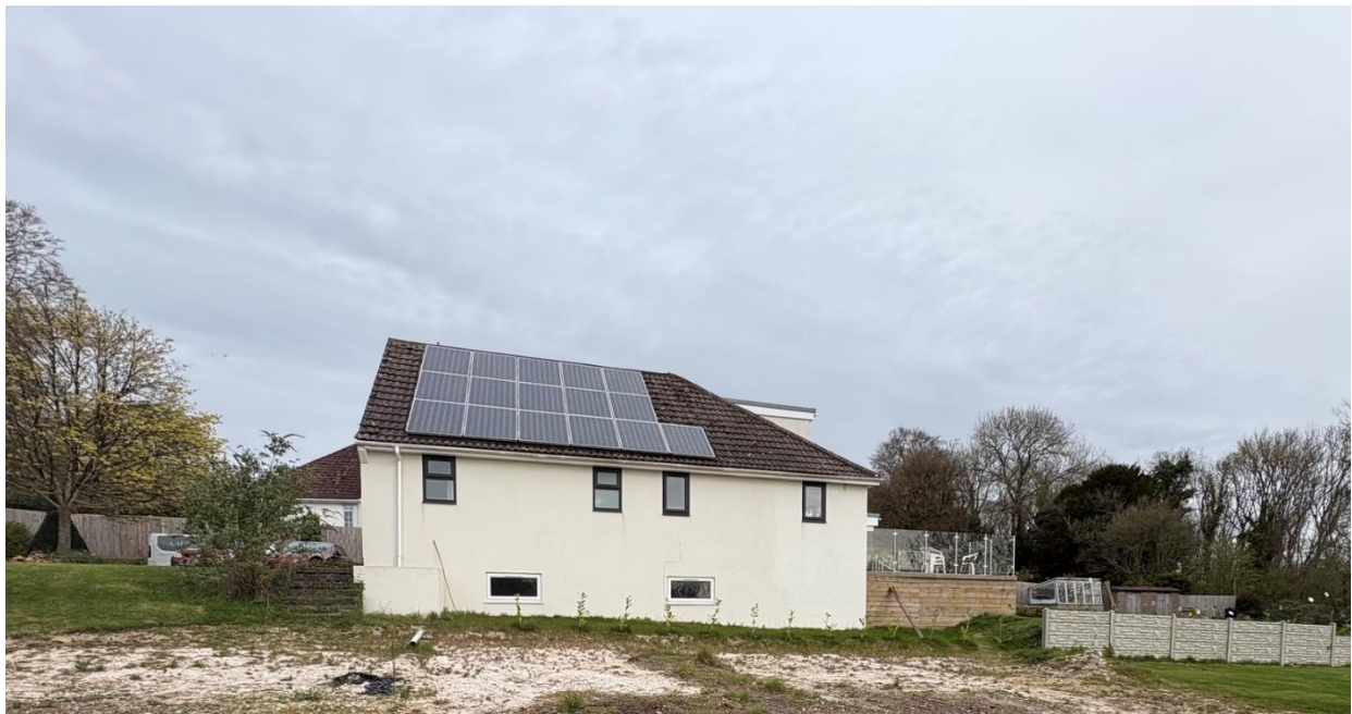
Side view of the Orchids which neighbours the site.
